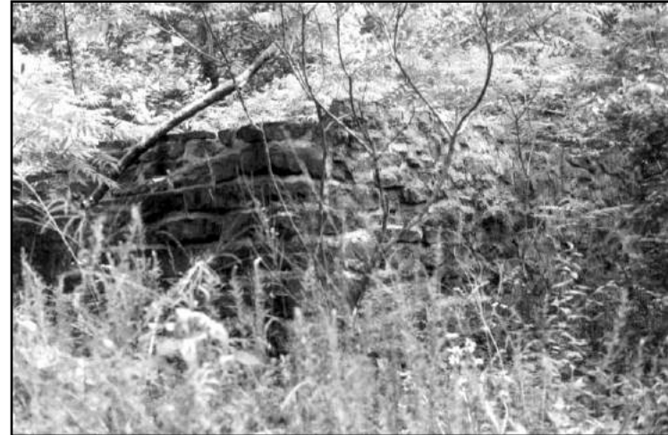
Figure 24: Whiteley School Foundations.
