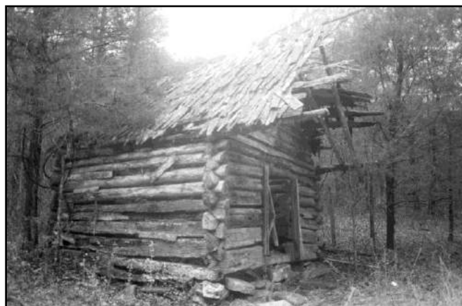
Figure 86: The Shake Roof Cabin was built of “recycled” logs.
