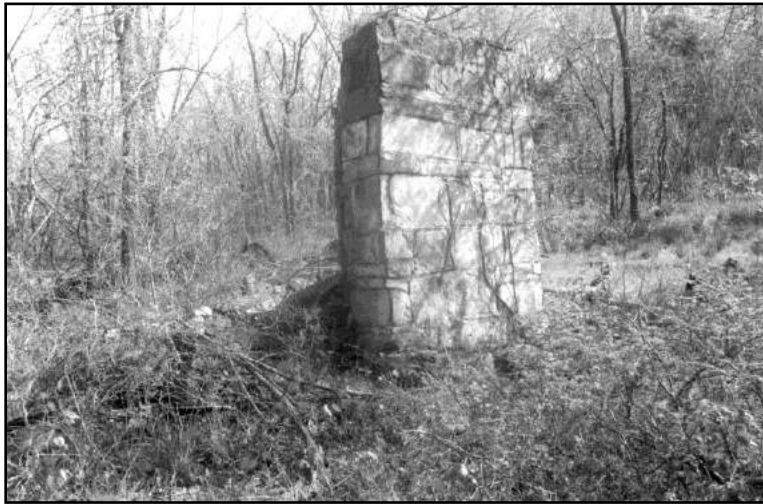
Figure 170: A portion of a chimney still stands at the house site on Tract 55-101.
