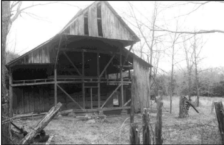
Figure 76: The large barn on the Farmer Farmstead has two interior log cribs.
