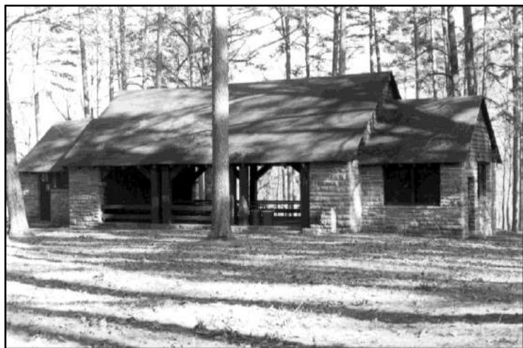
Figure 205: The CCC Picnic Pavilion at Buffalo River State Park.
