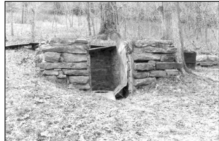
Figure 50: Granny Henderson's root cellar.
