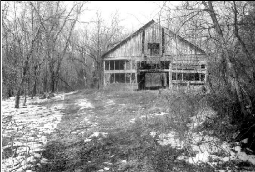
Figure 150: The barn on the Mays property has also deteriorated.
