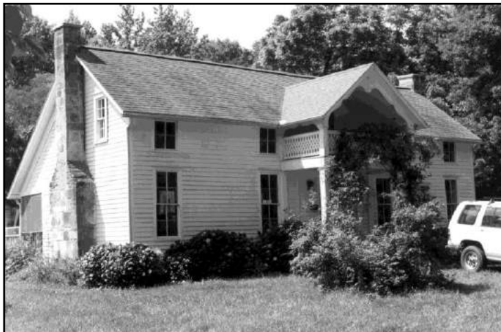
Figure 30: The Casey-Clark House.
