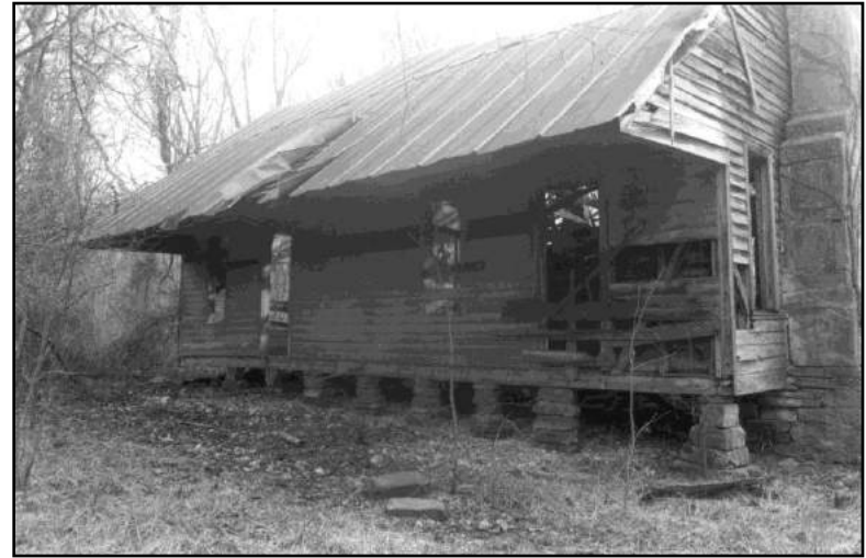
Figure 189: The A.G. Smith House is in ruins.
