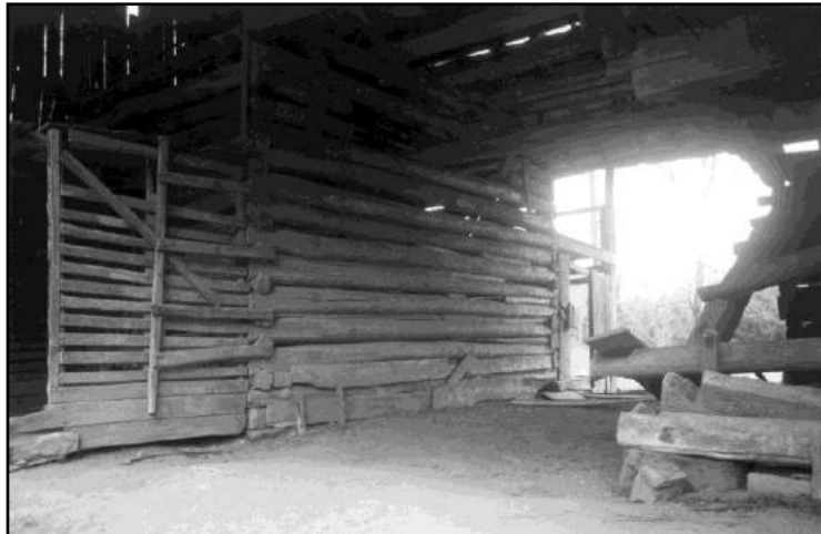
Figure 77: An interior view of the Farmer Barn showing the log crib construction.
