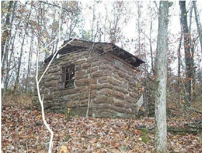
Figure 207: The CCC constructed utility building. ( Photo courtesy of Buffalo National River )
