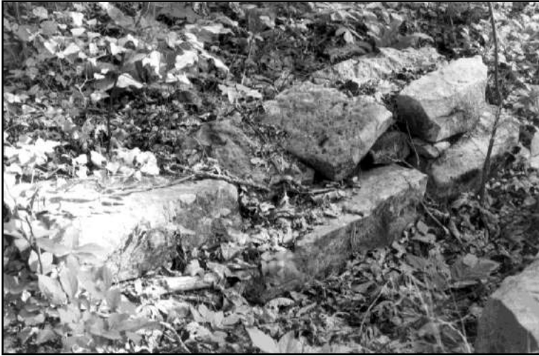
Figure 143: This tiered box vault grave in Deffenbaugh Cemetery has deteriorated substantially.
