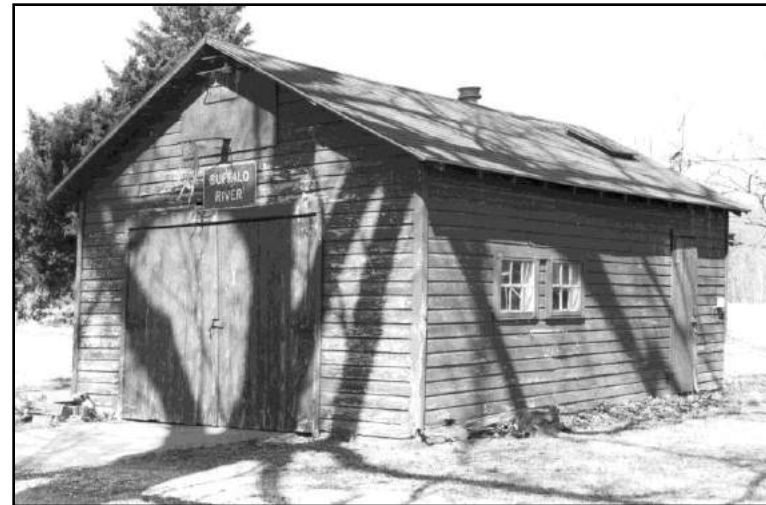
Figure 198: Garage on Tract No. 06-125.
