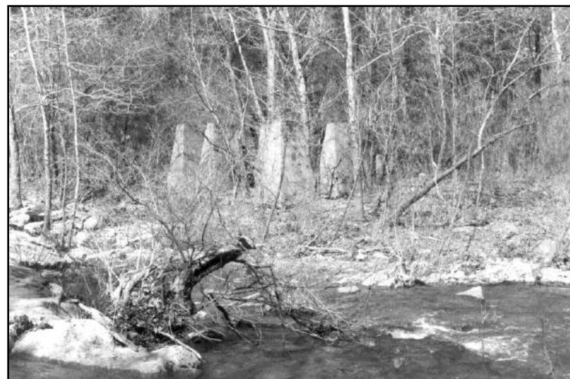
Figure 229: Concrete pilings stand on the northeast side of Clabber Creek.
