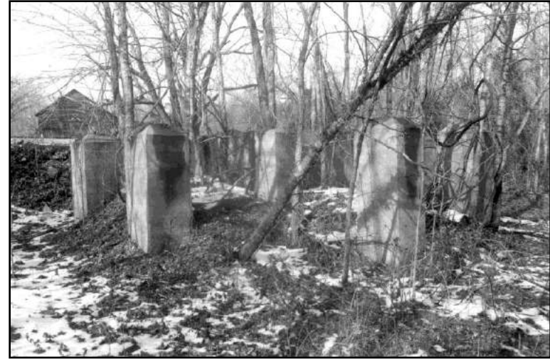
Figure 211: Concrete piers near the railroad grade at Gilbert.
