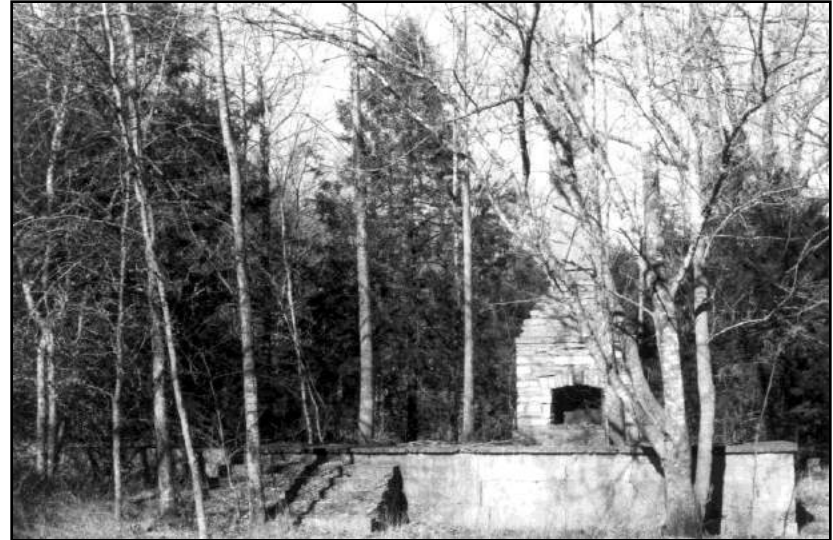
Figure 105: Foundations and chimney at the Angle House Site.
