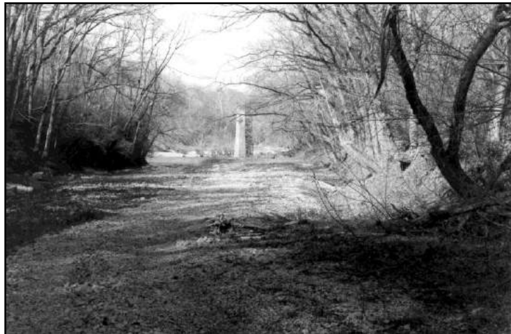
Figure 213: This view shows the railroad grade and bridge abutments looking north from the south side of the river.
