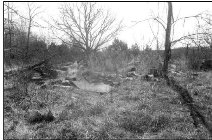
Figure 216: The Sanders House was destroyed by fire.
