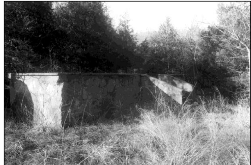
Figure 107: Remaining foundations at the McFadden House Site.
