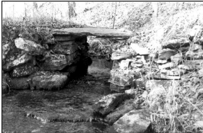
Figure 94: Rock bridge structure on the Huchingson property.
