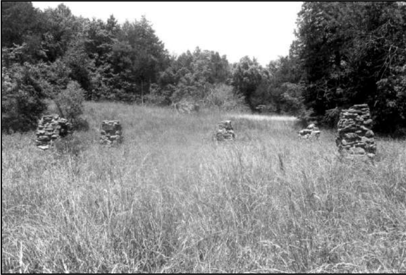
Figure 174: The stone piers of a turn-of-the-century cotton gin.
