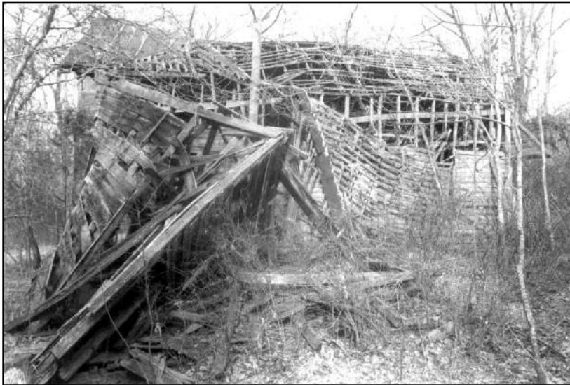
Figure 190: The A.G. Smith House rear façade.
