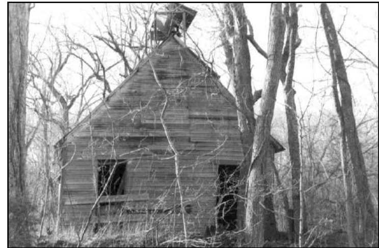
Figure 192: Main façade of Brown School.
