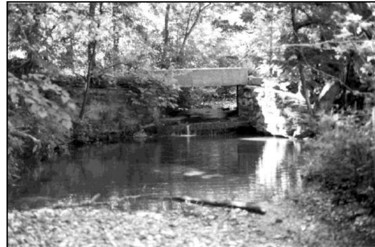
Figure 45: The Leatherwood Culvert in Boxley.
