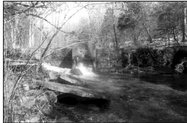
Figure 152: Mill Creek Dam-Lower View.
