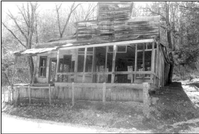
Figure 227: The Taylor-Medley Store in Rush is in poor condition.
