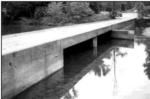
Figure 44: The Ponca Low Water Bridge.
