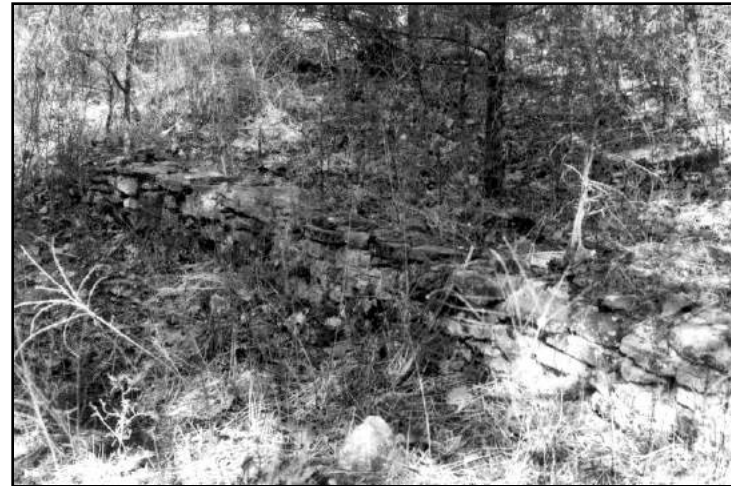
Figure 133: Dry Stack Stone Retaining Wall on Tract 12-107.
