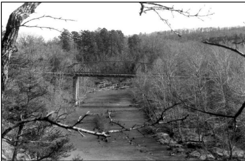
Figure128: The Highway 7 Bridge spans the Buffalo River.
