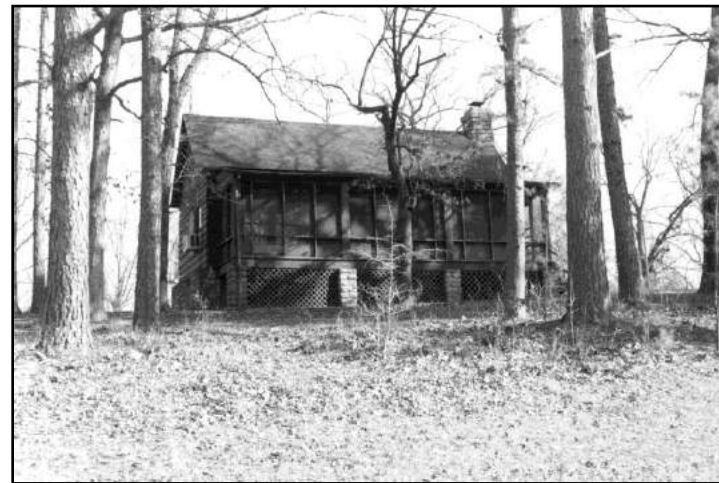
Figure 204: The cabins at Buffalo River State Park were constructed by the CCC.
