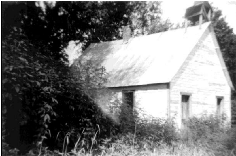
Figure 19: Brown School along Calf Creek was constructed ca. 1915. (Source: NPS, Buffalo National River .)
