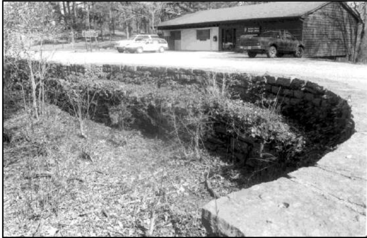
Figure 206: The CCC also constructed stone retaining walls at the Buffalo River State Park.
