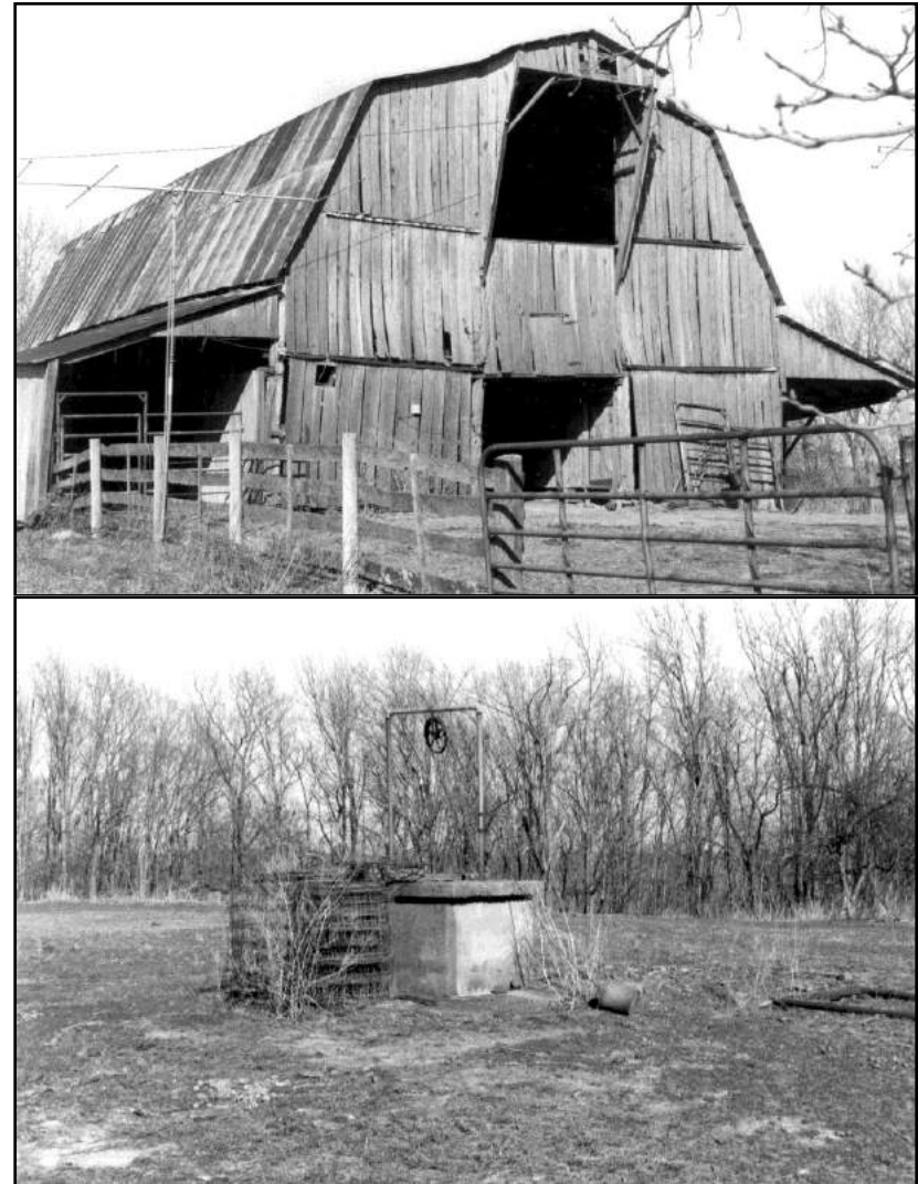
Figure 46: Remaining Barn and Well on Tract 65-109.
