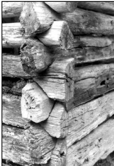
Figure 87: Detail of the log construction of the Shake Roof Cabin.
