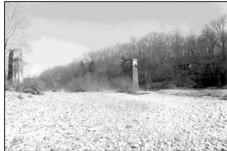
Figure 212: Railroad bridge abutments remain standing in the Buffalo River.
