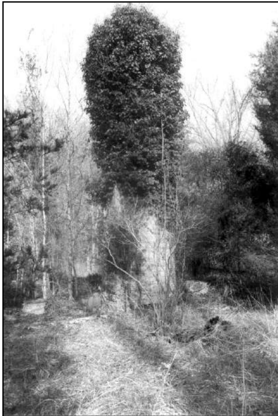
Figure 92: A stone chimney remains intact at the Huchingson House Site.
