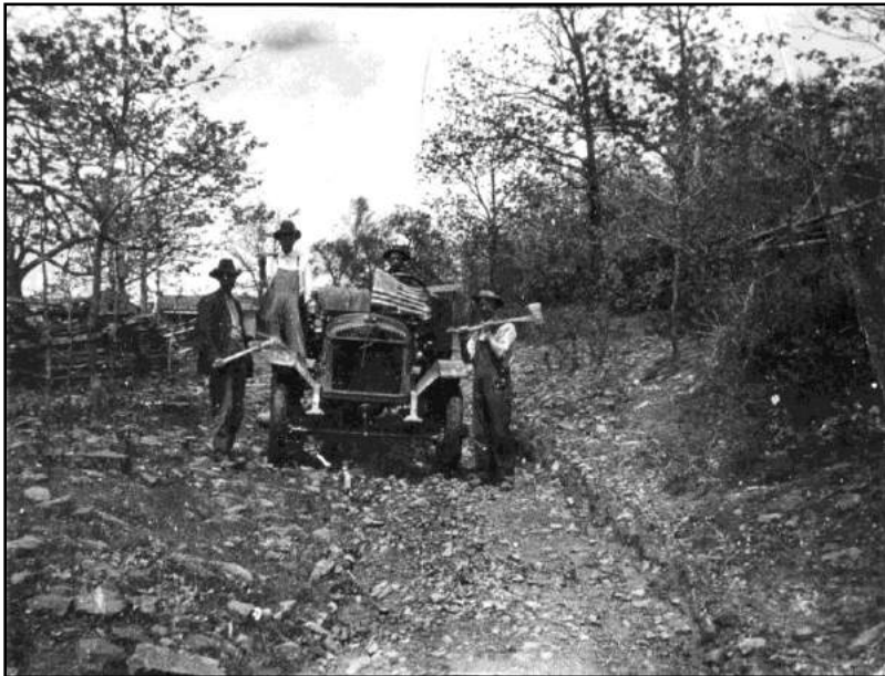
Figure 6: One of the first motorized vehicles in Newton County had to contend with rough and rocky unpaved roadbeds. (Source: NPS, Buffalo National River .)
