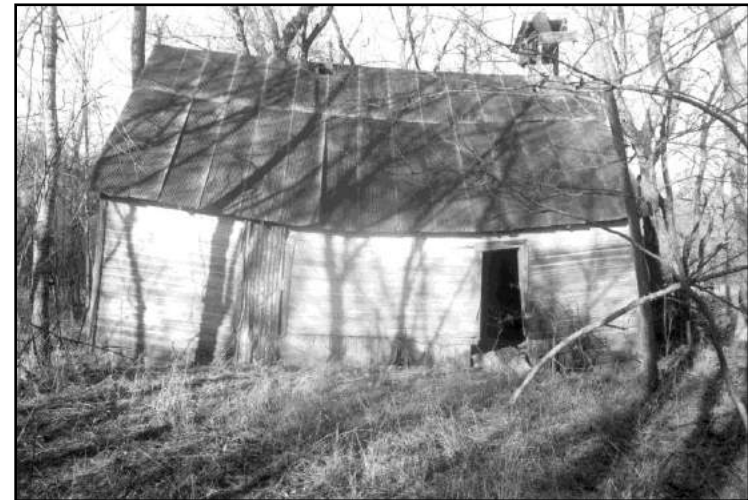
Figure 193: A side elevation of Brown School.
