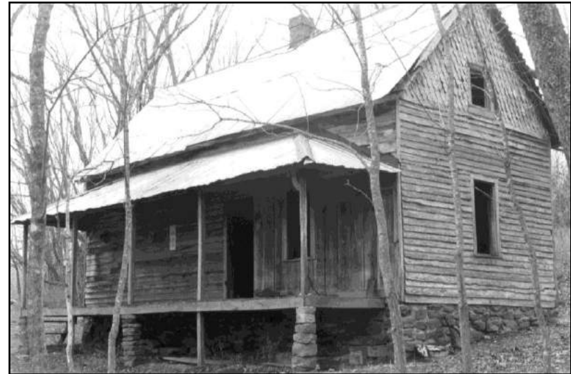
Figure 47: The Granny Henderson House.
