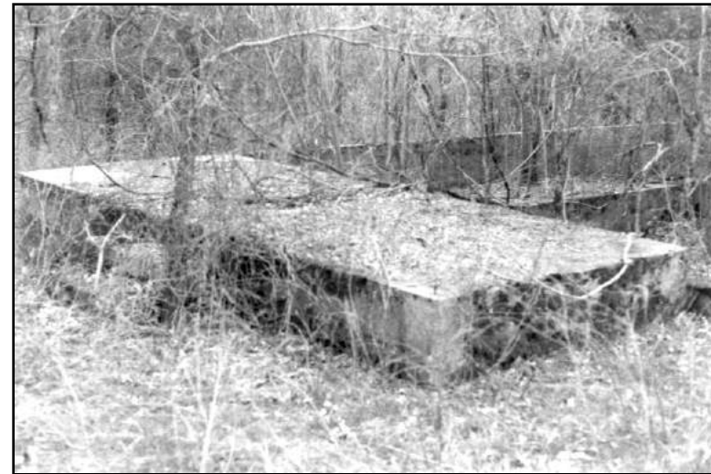
Figure 234: Concrete Foundation at House Site on Tract 77-417.
