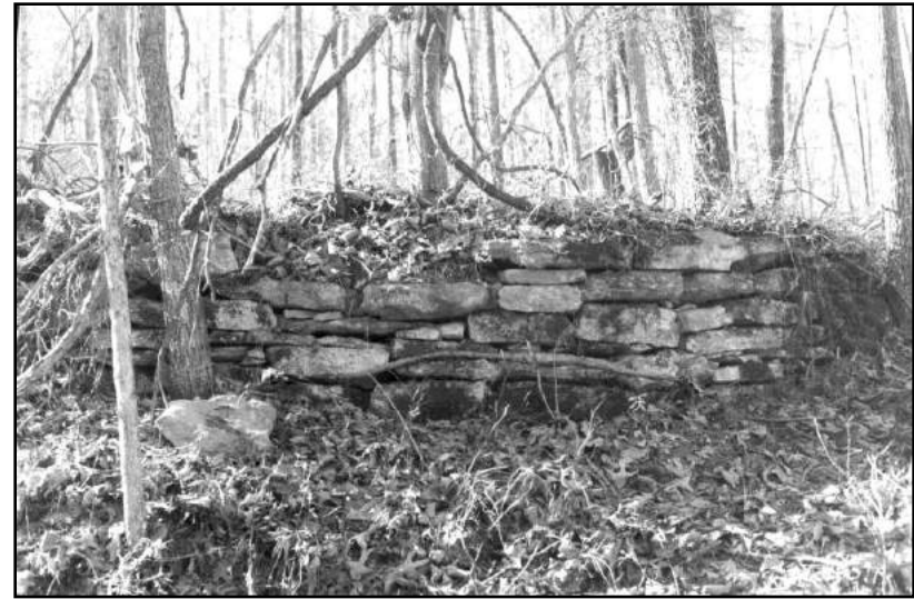
Figure 218: Dry Stack Stone Cistern located on the Ramsey Property.
