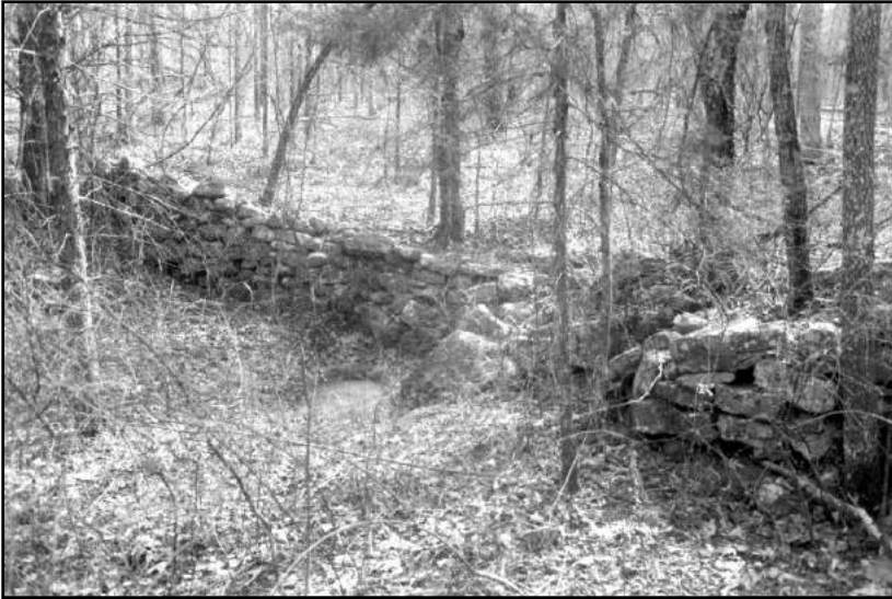
Figure 158: Dry Stack Stone Retaining Wall at John Reddell Property on Tract 59-101.
