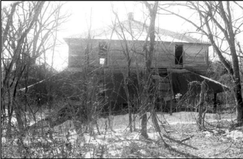
Figure 148: The Mays House has deteriorated significantly after several decades of disuse and neglect.
