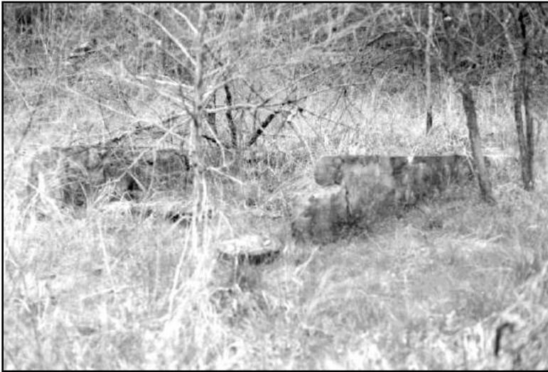
Figure 233: Garage Foundation at House Site on Tract 74-110.
