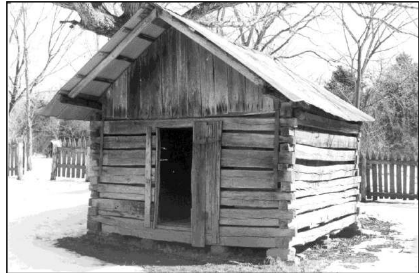
Figure 183: The log smokehouse on the Collier Homestead.
