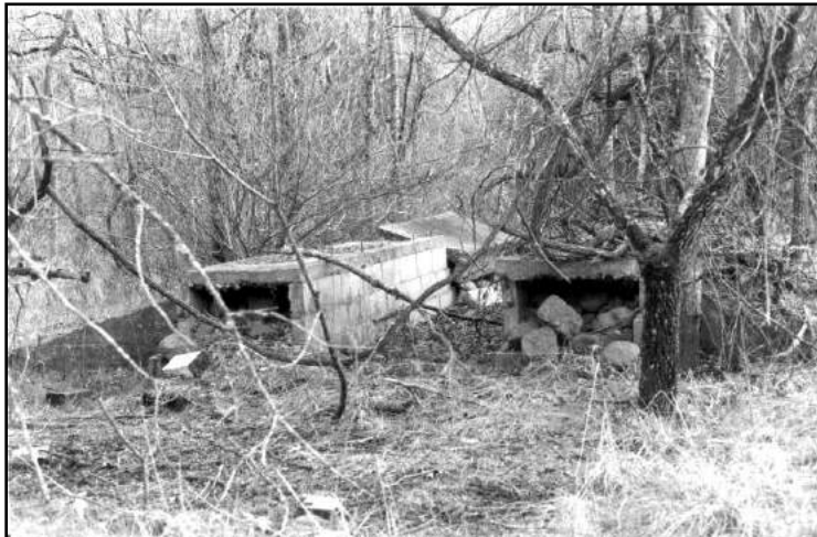
Figure 96: Remaining foundations of the Tinsley milkhouse.
