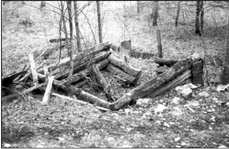
Figure 78: The log springhouse on the Farmer Farmstead has collapsed.
