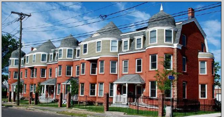
235-257 William Street. (Courtesy of Greta Bush and Habitat for Humanity of Coastal Fairfield County)
