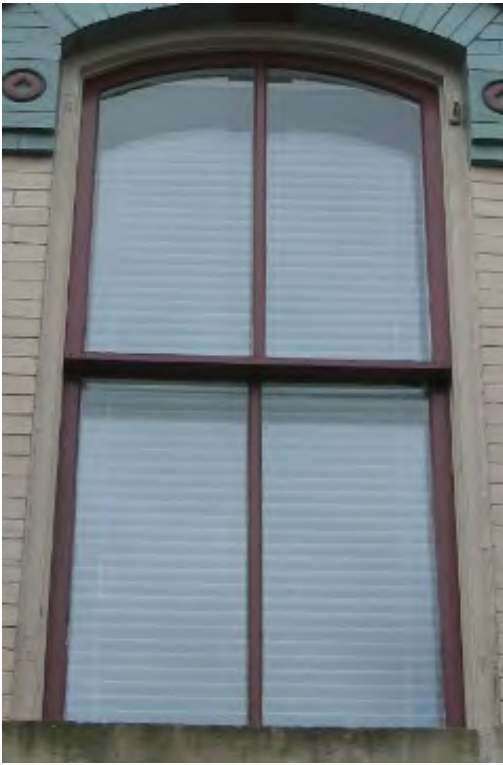
Original, two-over-two, wood sash window at 306 Centre Street.
