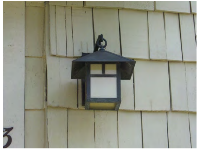
This new light fixture is an appropriate design for the style of the historic building at 326 South Seventh Street.
