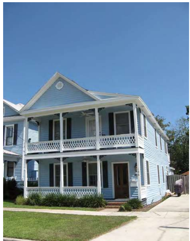
Gable front dwelling at 106 South Seventh Street.
