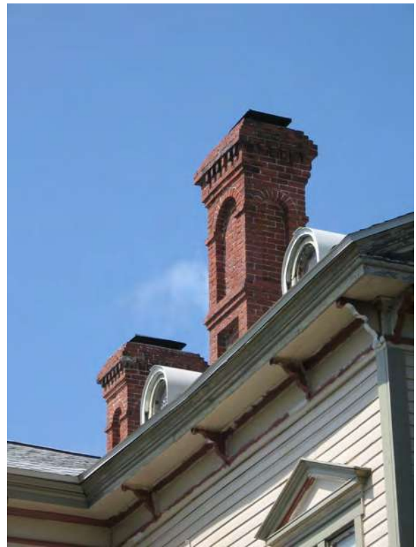
Chimneys with decorative corbelling and arched inset. (227 South Seventh Street)
