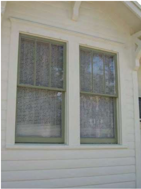
Original, three-over-one wood sash windows. (202 South Seventh Street)
