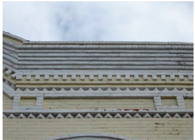
Preserve features like brick corbelling. (117 Centre Street)
