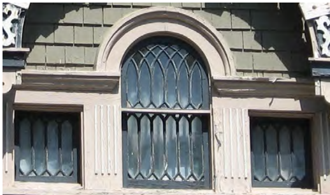
Palladian window at 130 South Seventh Street.
