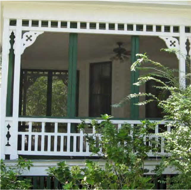
Detailed wood trim at 121 North Sixth Street.
