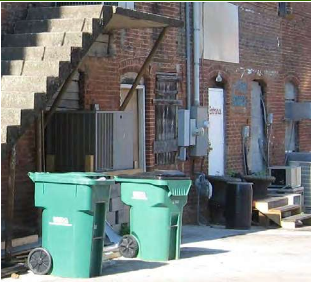
HVAC units, utility meters, and garbage containers are typically placed behind commercial buildings.
