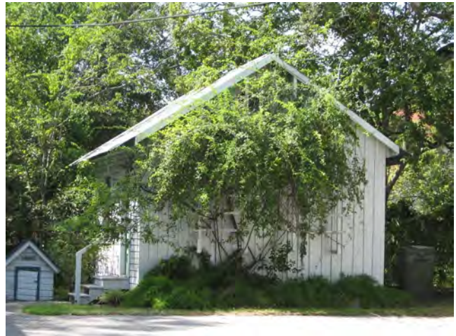
Well-maintained original outbuilding at 121 North Sixth Street.
