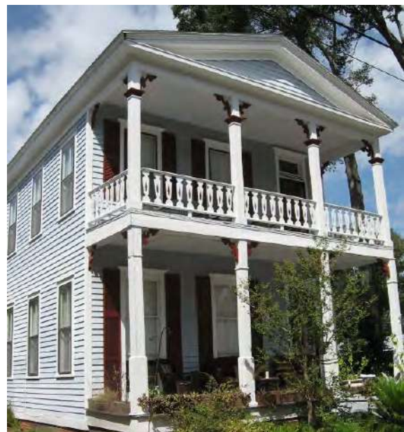
Follow the guidelines above for wood siding like those on the dwelling at 111 South Fifth Street.
