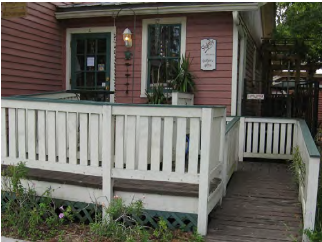
The handicapped ramp at 218 Ash Street blends into the existing porch and railing.
