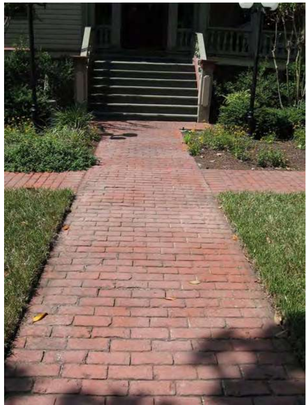
New walkways should be of brick or patterned concrete such as at 227 South Seventh Street.
