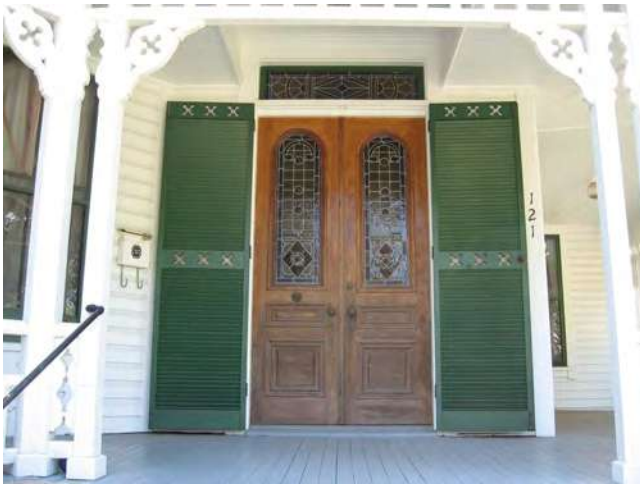
Wooden trim and other traditionally painted building elements should be kept painted. (121 North Sixth Street)
