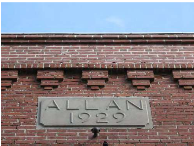
The brick building at 309-311 Centre Street has decorative brick corbelling and a concrete name – and date-stone inset, which should be maintained and preserved.
