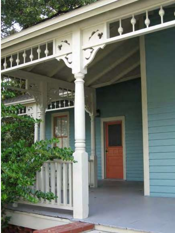
Porch elements are character-defining features and should be preserved and maintained. (28 North Fourth Street)
