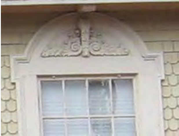
The highly detailed decorative trim in this window hood should be maintained and preserved. (315 Alachua Street)
