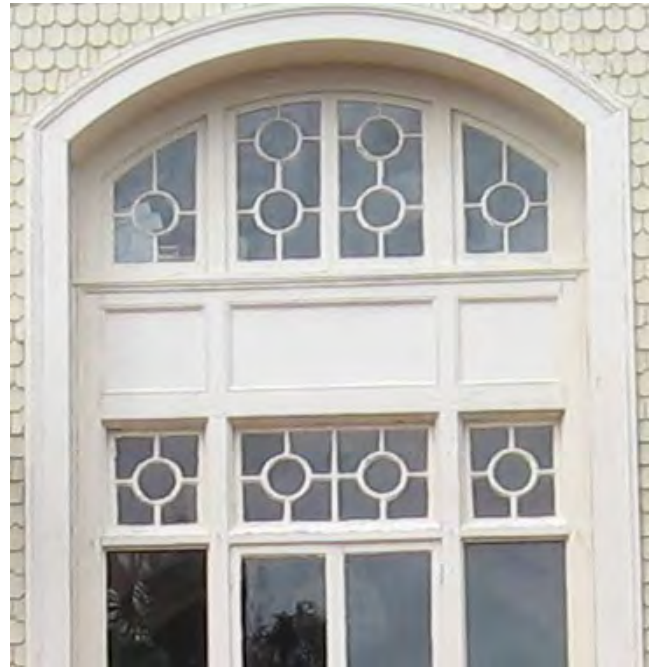
Some windows were designed to be essential parts of a dwelling's character. (315 Alachua Street)
