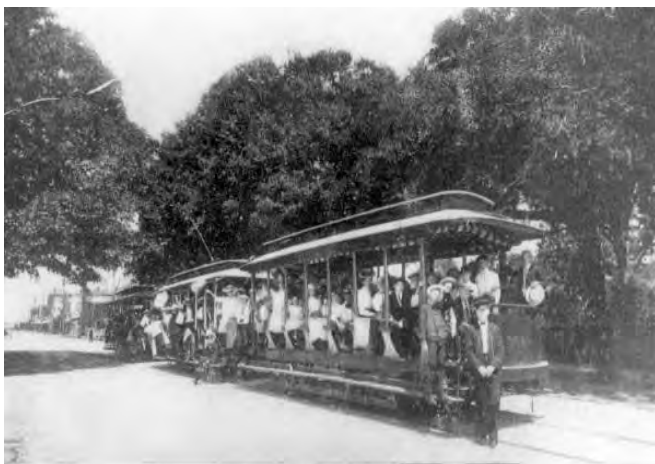
Streetcar tracks were installed around the turn of the twentieth century. (Photo courtesy of the Florida State Library and Archives)
