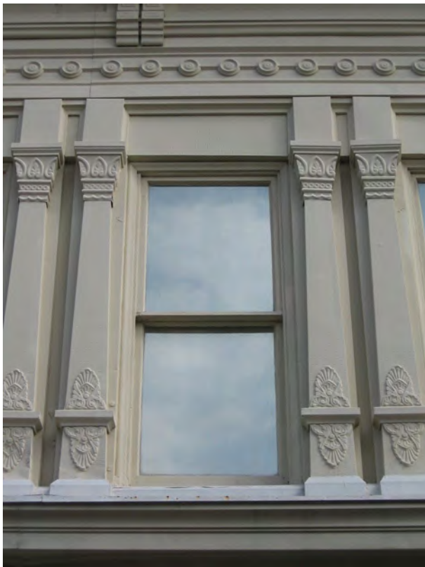
One-over-one wood sash window at 313-319 Centre Street.
