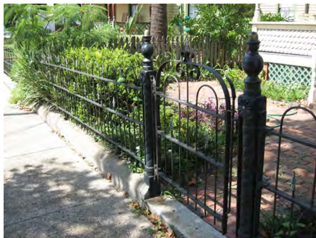
This original hoop and dart iron fence should be preserved. (605 Ash Street)
