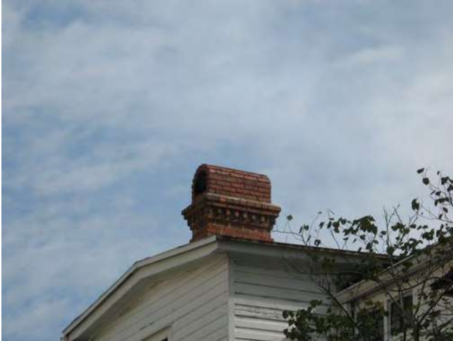
Decorative corbelled brick chimney with rounded cover pot at 415 Centre Street.
