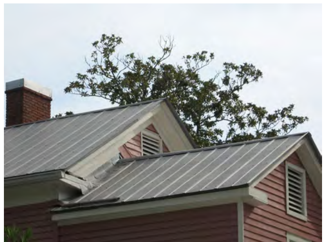
If a metal roof must be replaced, the replacement should match the historic one as closely as possible. (218 Ash Street)
