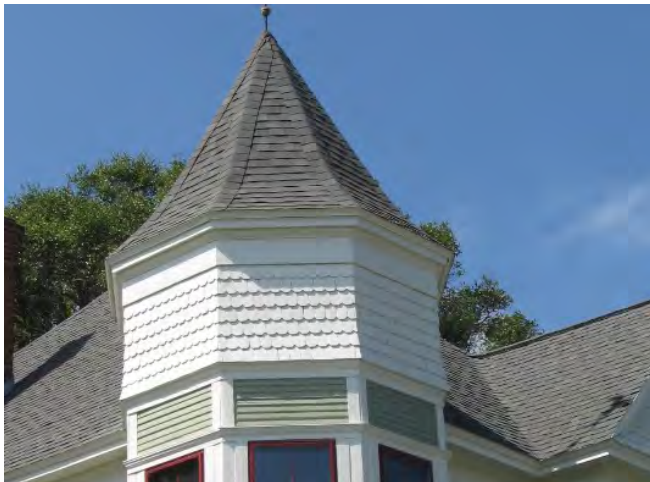
A complex, irregular roof is a crucial stylistic element of the Queen Anne house; it should be retained and kept in good repair. (117 North Sixth Street)
