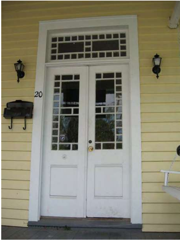
This entrance, with original multi-light wood panel double doors and transom, enhance the character of the house and should be preserved. (20 South Fourth Street)
