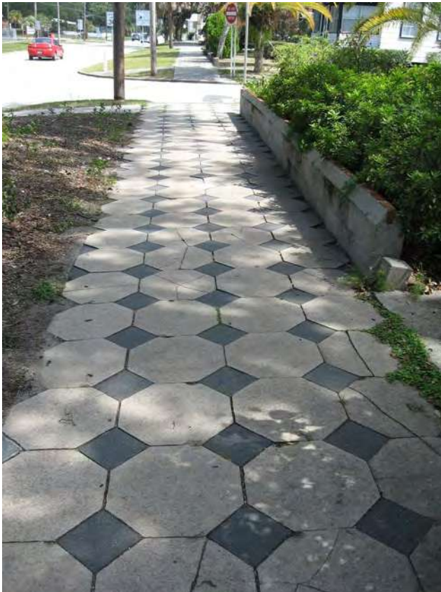
Historic walkway surface in the 800 block of Atlantic Avenue.
