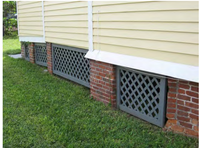
Lattice panels can be appropriate in terms of design and installation, though should be cut to fit in between foundation piers, as these custom panels do, rather than conceal or cover them. (20 South Fourth Street)
