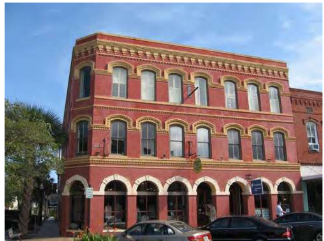
The Hoyt Building at 201-203 Centre Street was built in 1876.
