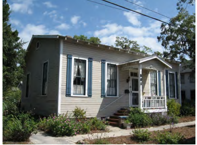
This side-gabled dwelling at 501 Beech Street is reflective of the simple house forms in the historic district which can be characterized as vernacular.
