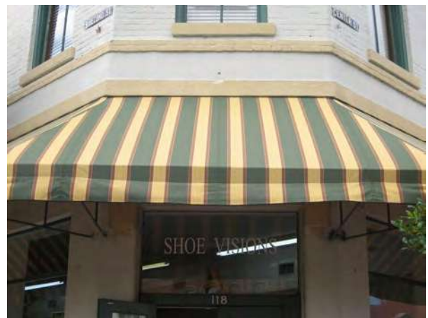
The canvas shed awning is appropriately shaped to follow the contour of the building's chamfered corner. (118 Centre Street)
