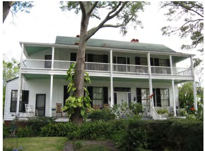
The Lesesne House at 415 Centre Street is illustrative of the city's historic architecture.
