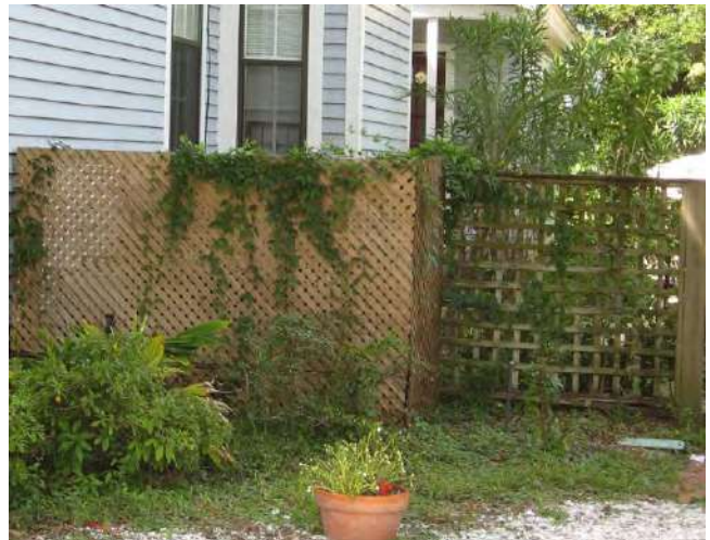
Screening a HVAC unit reduces its visual effect while still allowing for access. (111 South Fifth Street)
