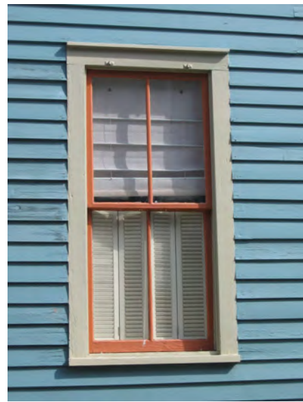
Original two-over-two wood sash windows. (28 North Fourth Street)
