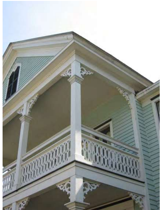
Paint helps protect wooden elements from decay. (614 Ash Street)
