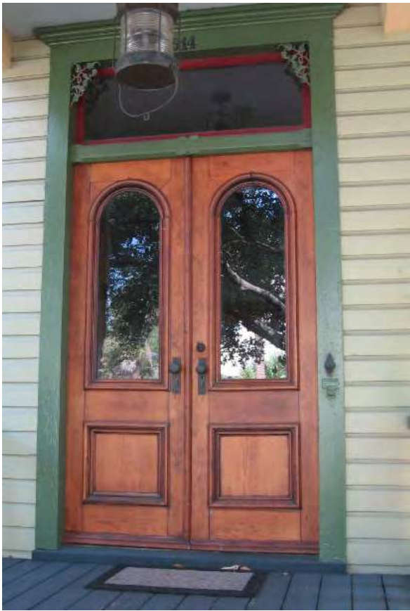
Original arched-light doors and transom at 614 Beech Street.
