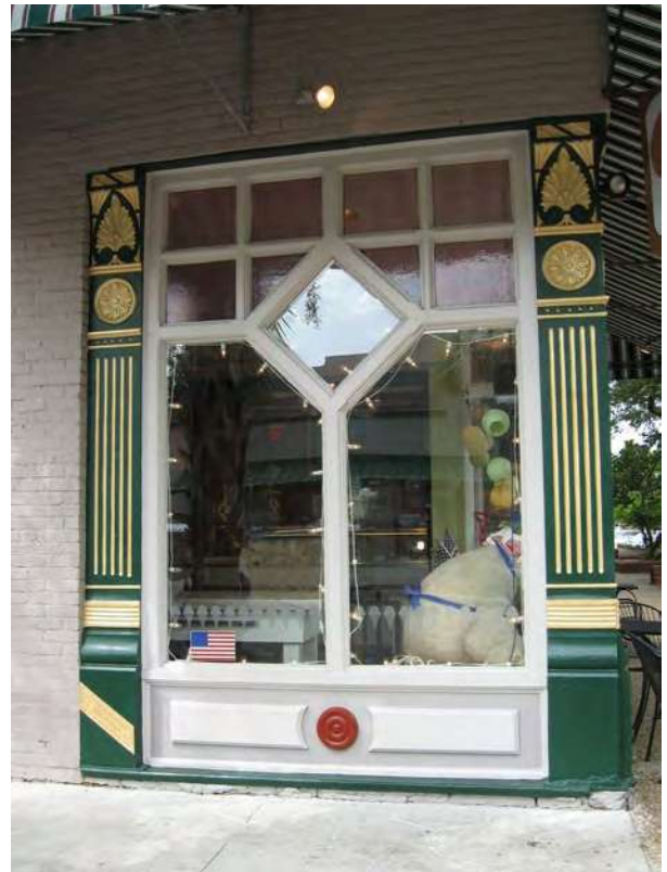
This storefront at 218 Centre Street retains original elements including bulkheads and display windows.
