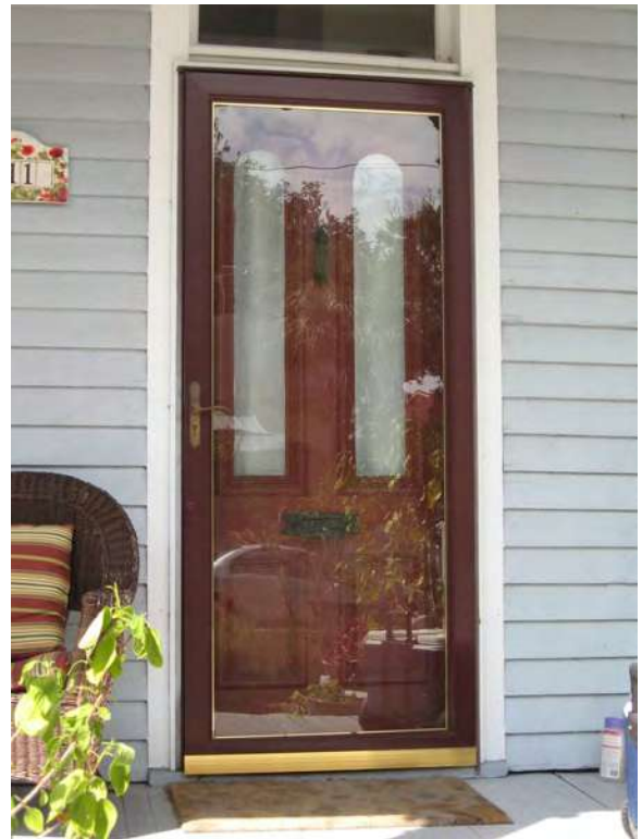
This original two-arched-light door at 111 South Fifth Street is a character-defining feature and should not be obscured. It has a storm door that appropriately allows a full view of the door.
