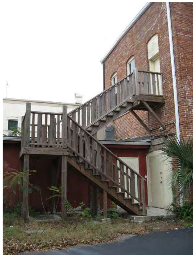
This fire escape is an appropriate model due to its location at the rear elevation and simple wood construction. (313 Centre Street)
