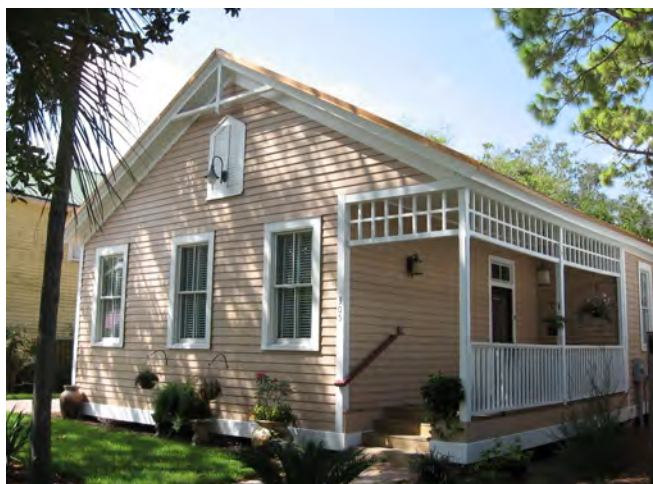
Rehabilitated dwelling at 305 South Sixth Street.
