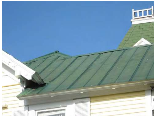
Keep metal roofs painted. (305 South Eighth Street)
