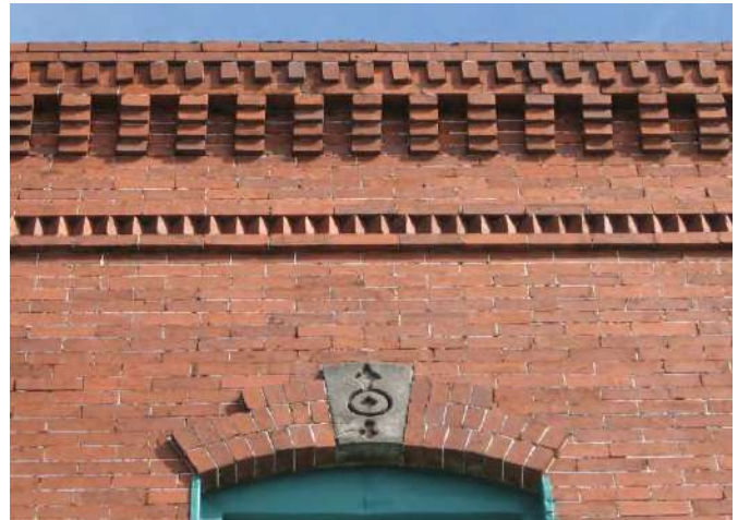
Unpainted masonry surfaces can be important aspects of character and should remain unpainted. (215-217 Centre Street)
