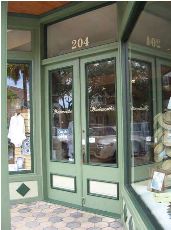
Painted surfaces should be maintained, as at 204 Centre Street.
