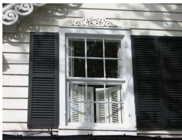
Six-over-six wood sash windows and appropriate shutters. (15 North Fourth Street)
