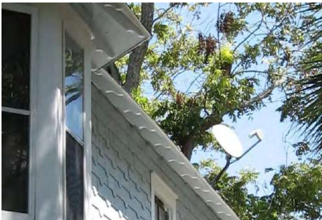
The placement and size of this dish at the rear elevation helps minimize its visual impact on the dwelling. (214 South Seventh Street)
