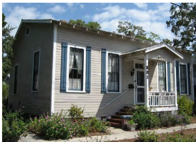
An existing building represents embodied energy. (501 Beech Street)
