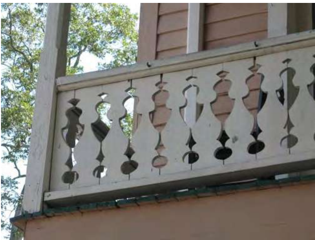
This type of detailed porch railing can be found on some Folk Victorian dwellings. (322 S. Sixth Street)
