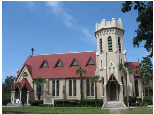
St. Peter's Church at 801 Atlantic Avenue exemplifies the Gothic Revival style.
