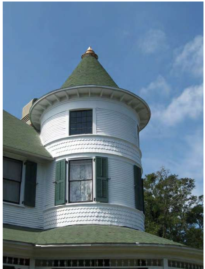
The corner tower is a dominant feature of the Queen Anne-style Waas House at 327 South Seventh Street.
