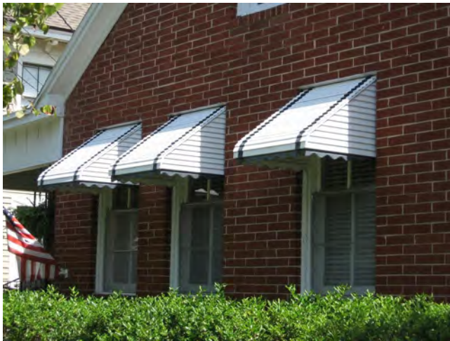
These shed-type awnings are appropriately installed one over each individual window; do not install a single awning that covers wall surface between windows. (306 South Seventh Street)
