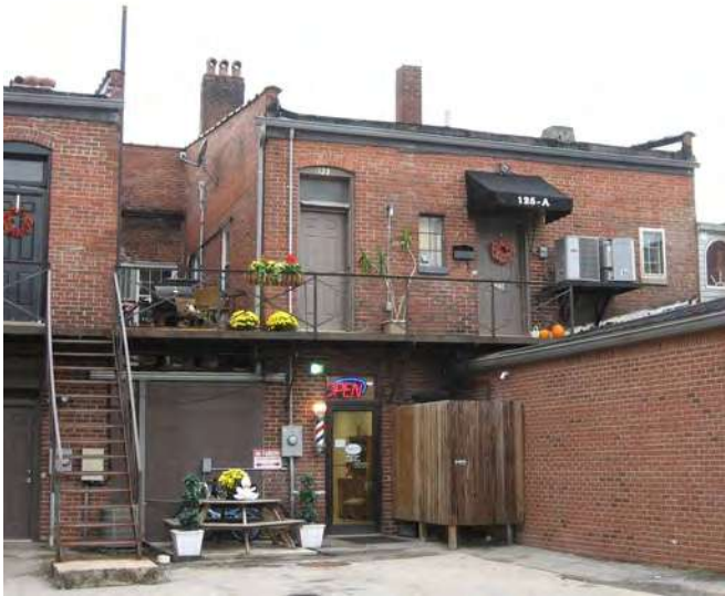
Rear decks can be used to tie buildings together and access upper floor space.
