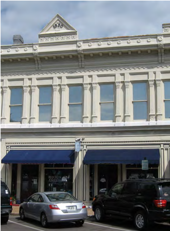
Metal façade at 313-319 Centre Street.
