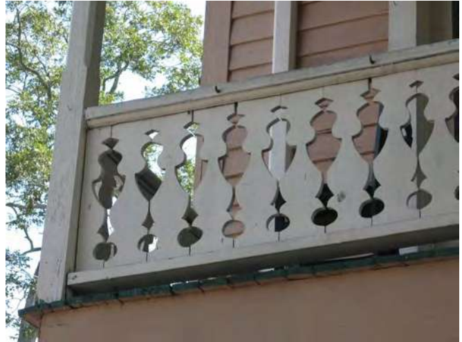
The milled wood porch railing should be maintained and preserved, as at 322 South Sixth Street.
