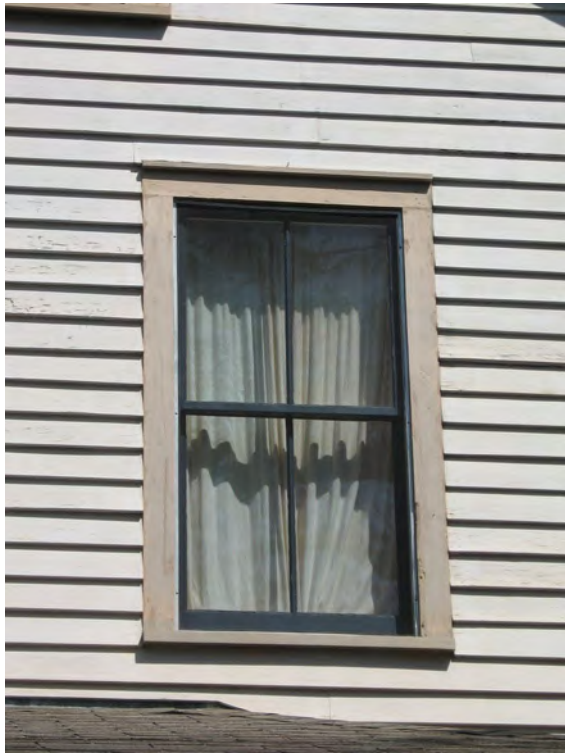
The design of this storm window allows for full view of the historic two-over-two, wood sash window behind it. (509 Beech Street)
