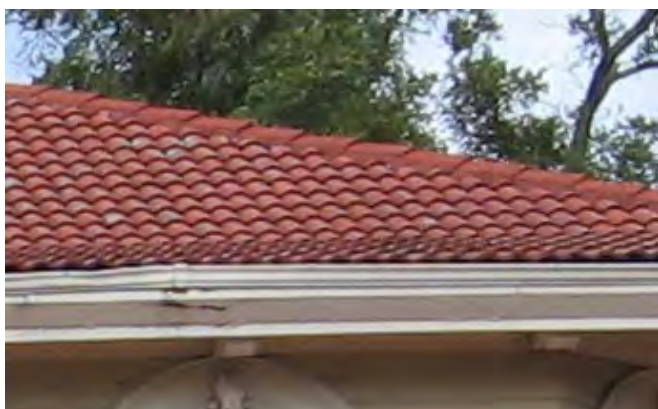
Retain and preserve original roof materials such as fired clay tile. (315 Alachua Avenue)
