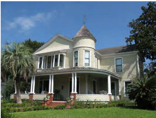
The Baker House at 112 North Sixth Street is a notable example of the Queen Anne style and features a wrap-around porch, corner tower, and asymmetrical plan.
