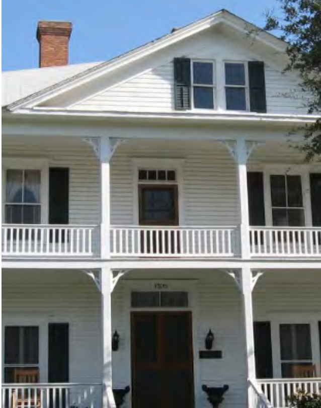
Original wood siding on the Oxley-Heard House.
