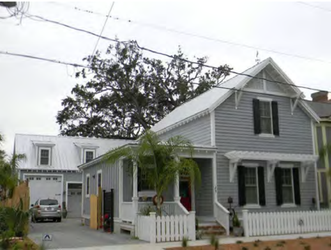
Example of infill which is compatible through its height, use of materials, window and door arrangement, and porch on the main façade. (23 South Sixth Street).
