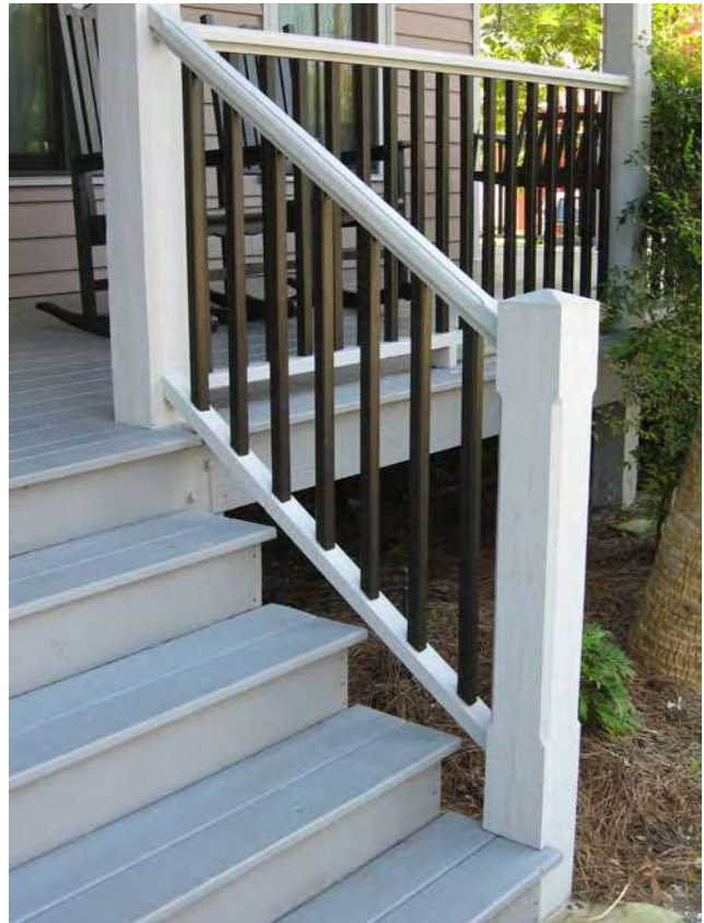
An appropriate example of rebuilt porch stairs at 604 Ash Street.
