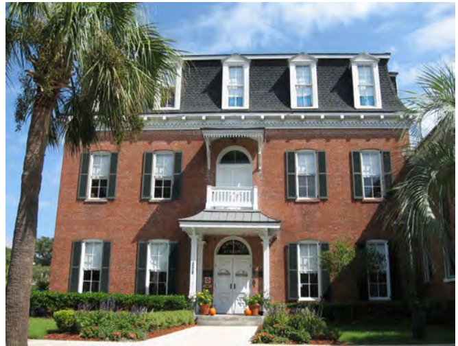
St. Michael's Academy at 505 Broome street is an example of the Second Empire style.
