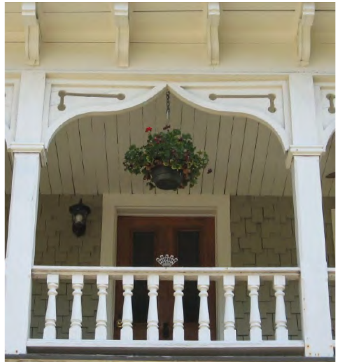
Eave brackets, balusters, and porch trim help convey a building's architectural style and contribute to its integrity. (302 South Seventh Street)
