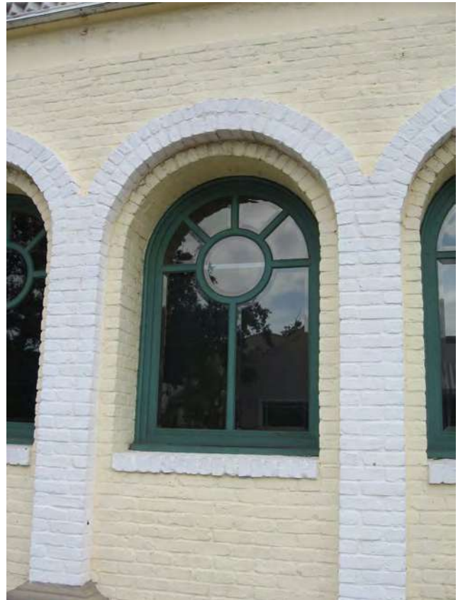
Distinctive arched storefront windows at 117 Centre Street.
