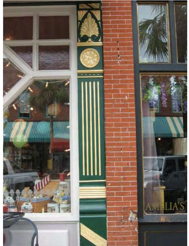
Cast iron features at 218 Centre Street are important elements of 19th century commercial buildings.
