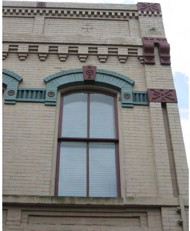
The exterior of the building at 306 Centre Street has extensive brick detailing, including the addition of color, which helps convey the architectural integrity of the building.
