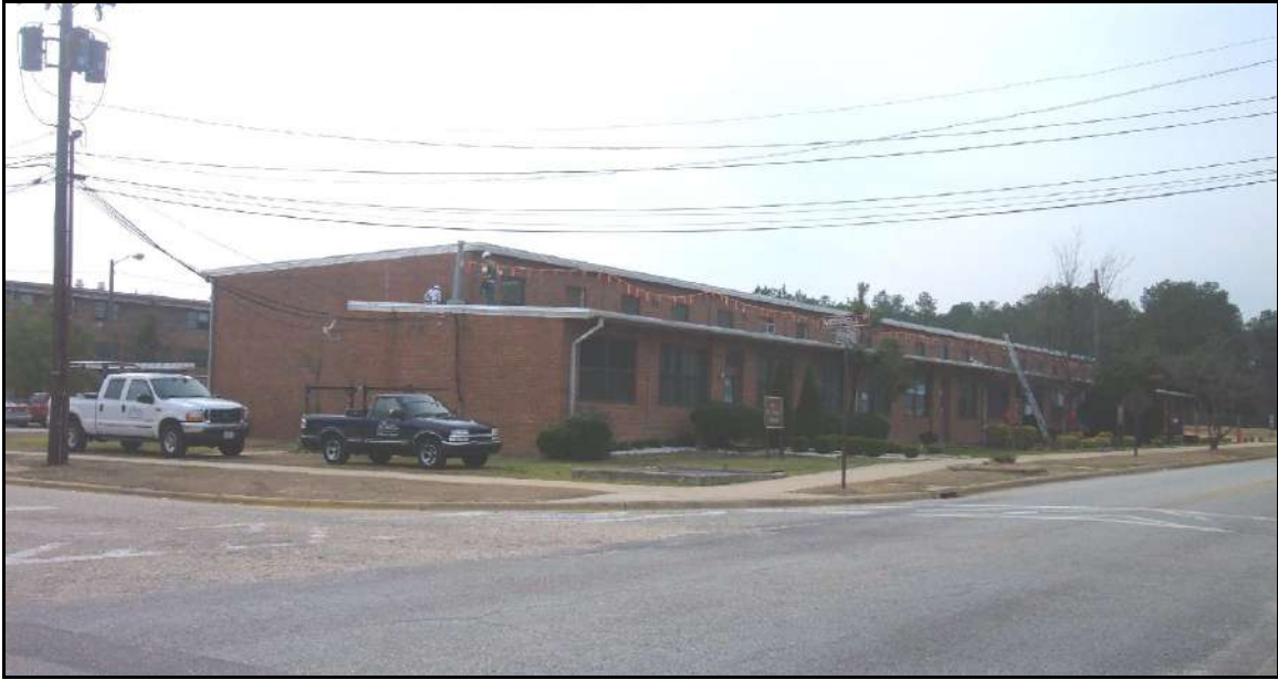
Building D-3225, north and west elevations.
