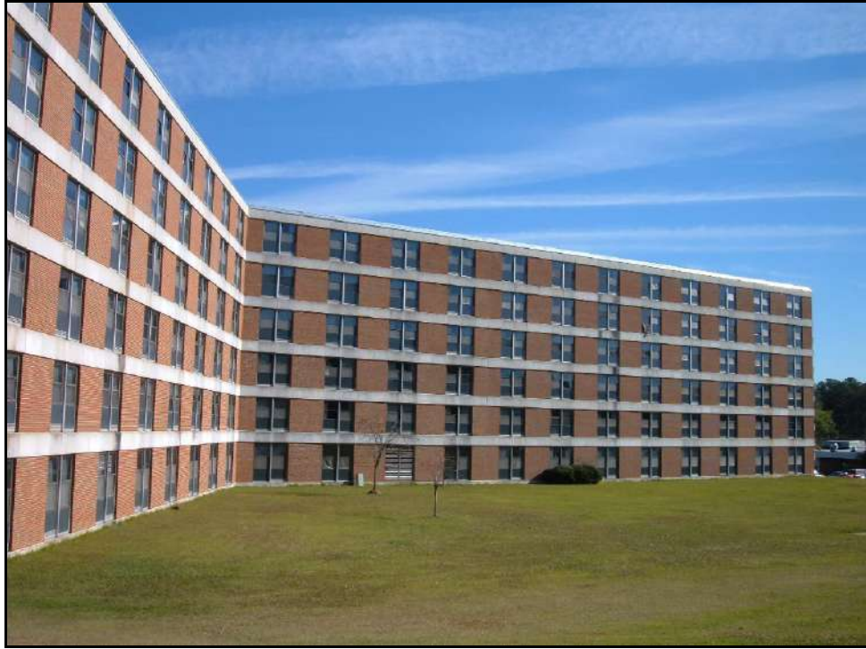
Building D-3705, west elevation.
