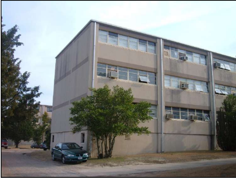
West and north elevations of Building C-6525.
