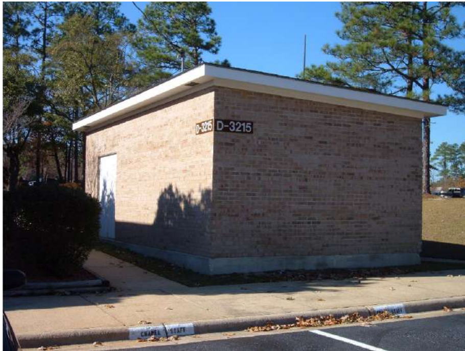
Figure 23: Building D-3215, south and east elevations. This building is located to the rear of the John F. Kennedy Memorial Chapel.
