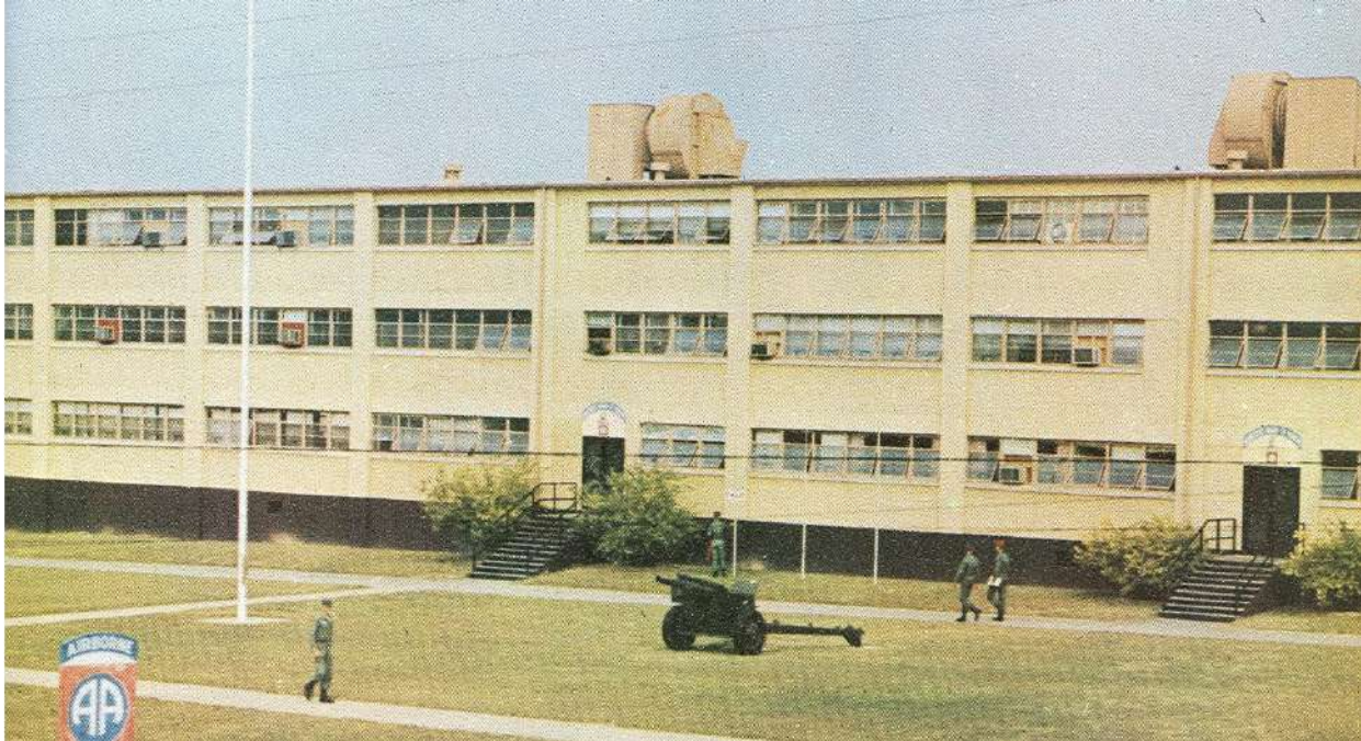
Building C-6525 in 1960, (Photo courtesy of the 82 nd Airborne Division Museum).
