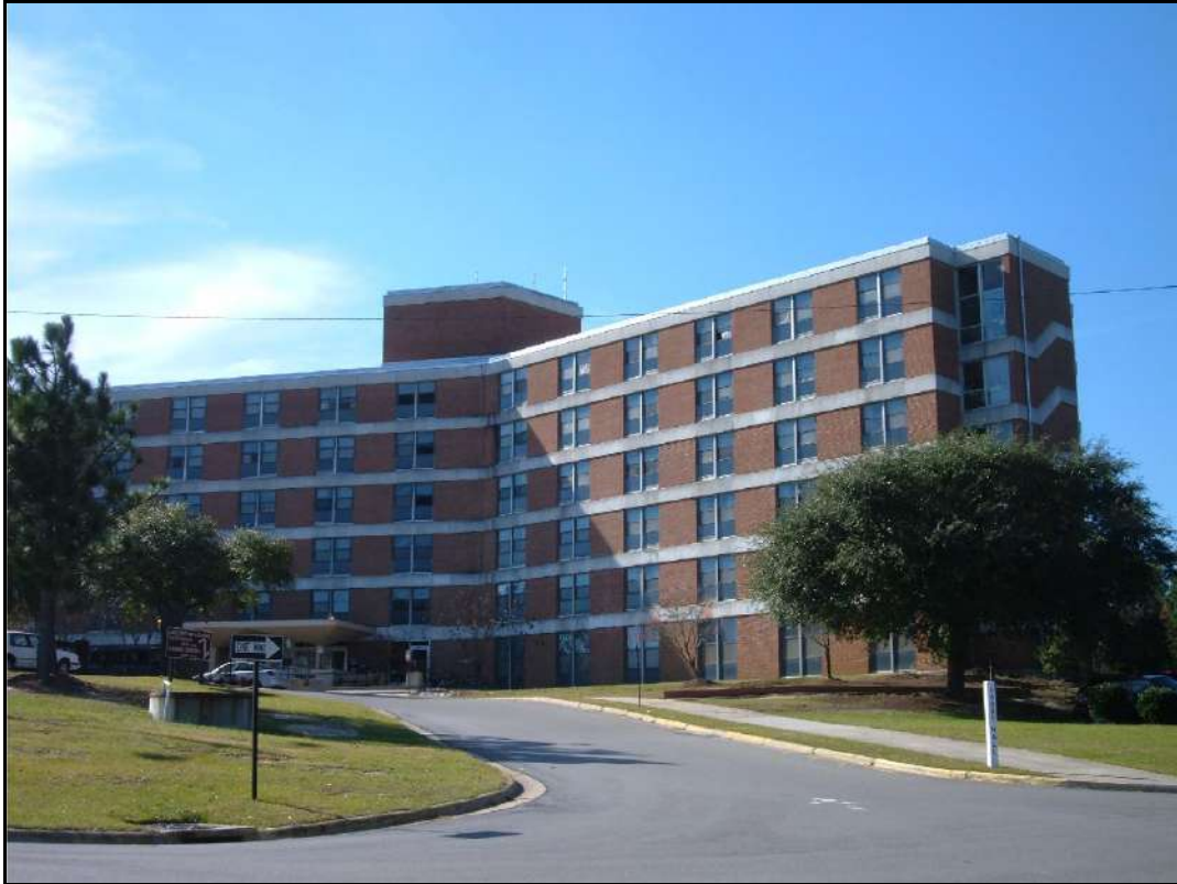
East and north elevations of Building D-3705.
