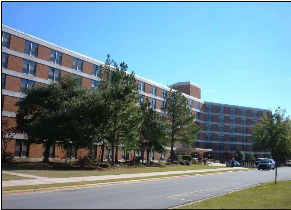
West elevation of Building D-3601.
