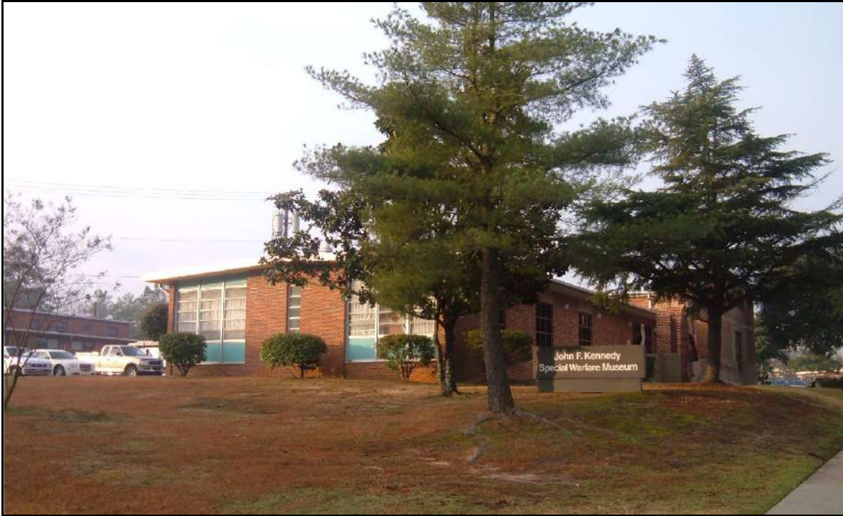
Building D-2502, north and east elevations.
