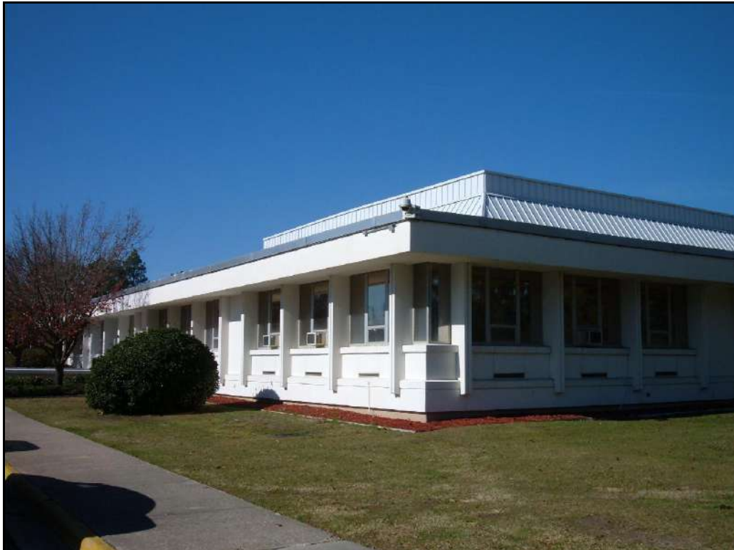
Figure 13: Kennedy Hall, south and east elevations.
