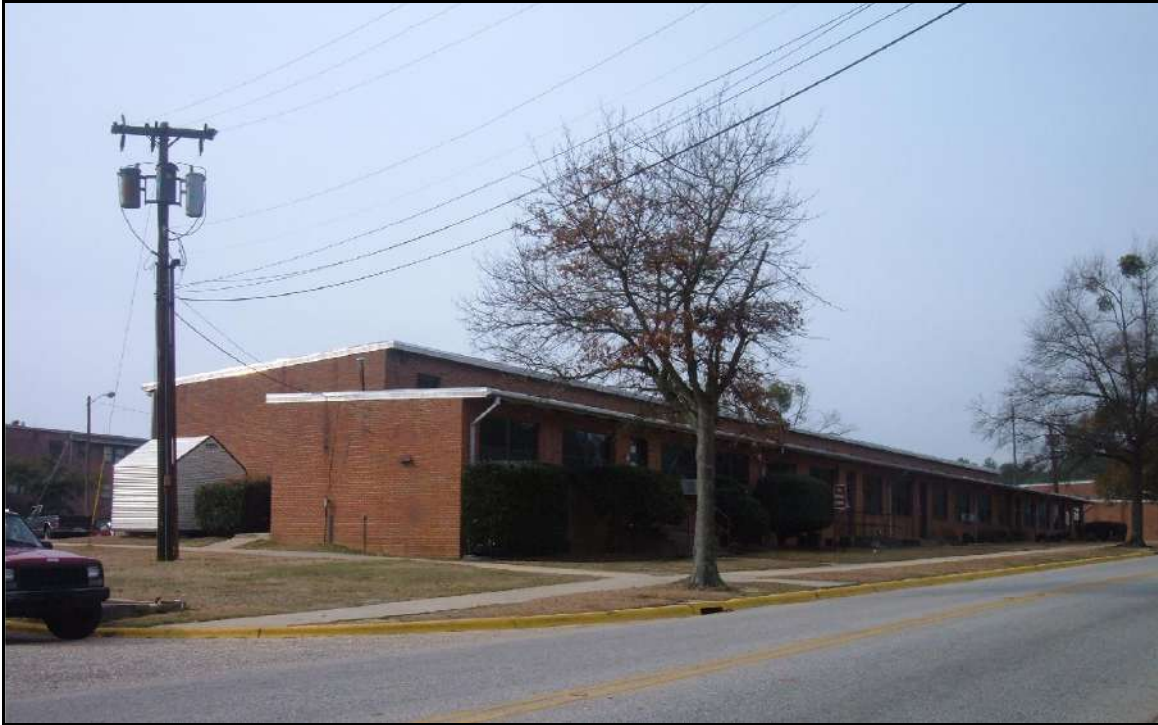
Building D-3022, north and east elevations.
