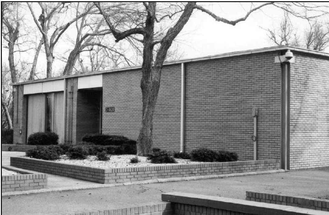
West elevation of Ridgway Hall.
