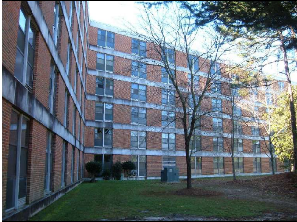
East elevation of Building D-3601.
