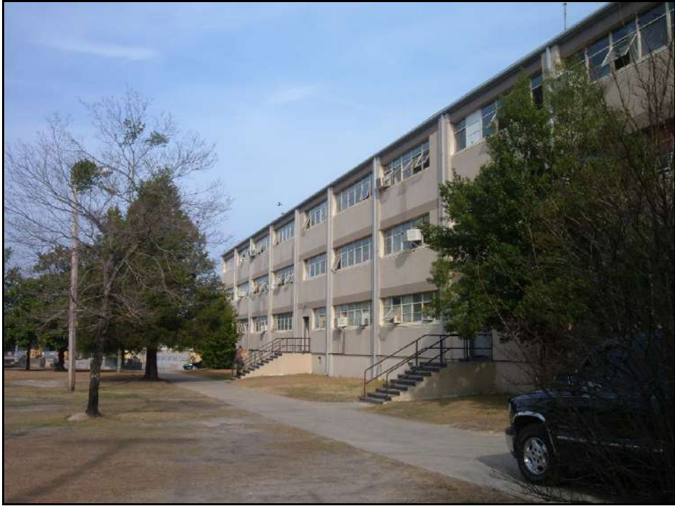
Building C-6525, west façade.
