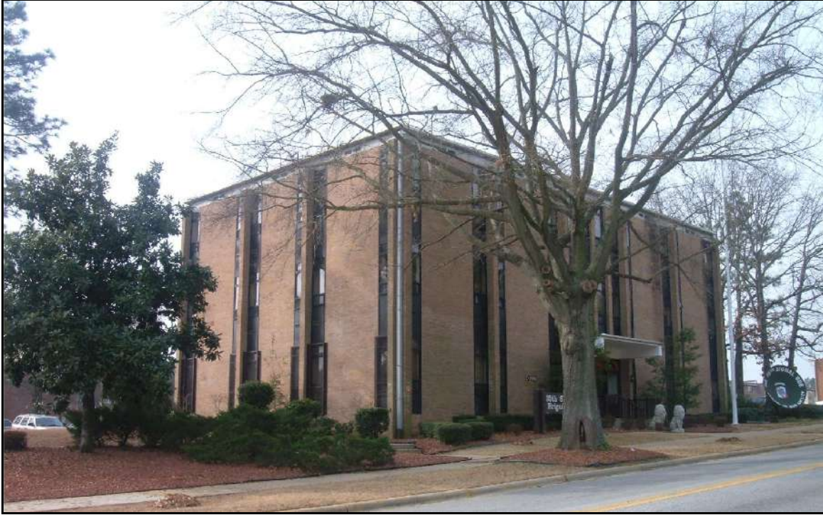
Building D-2919, north and east elevations.
