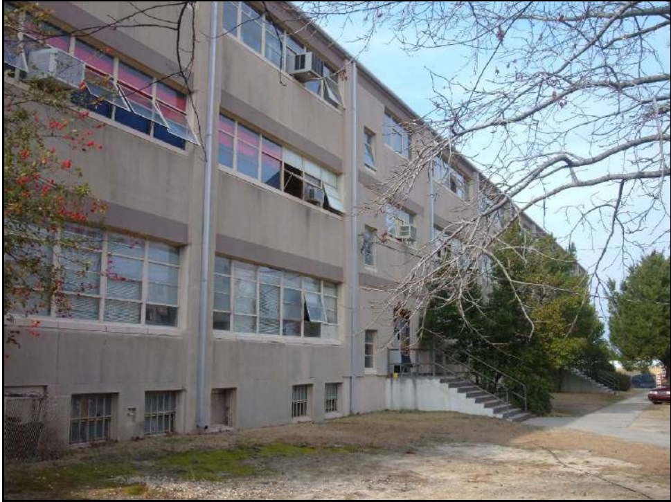
East elevation of Building C-6525.
