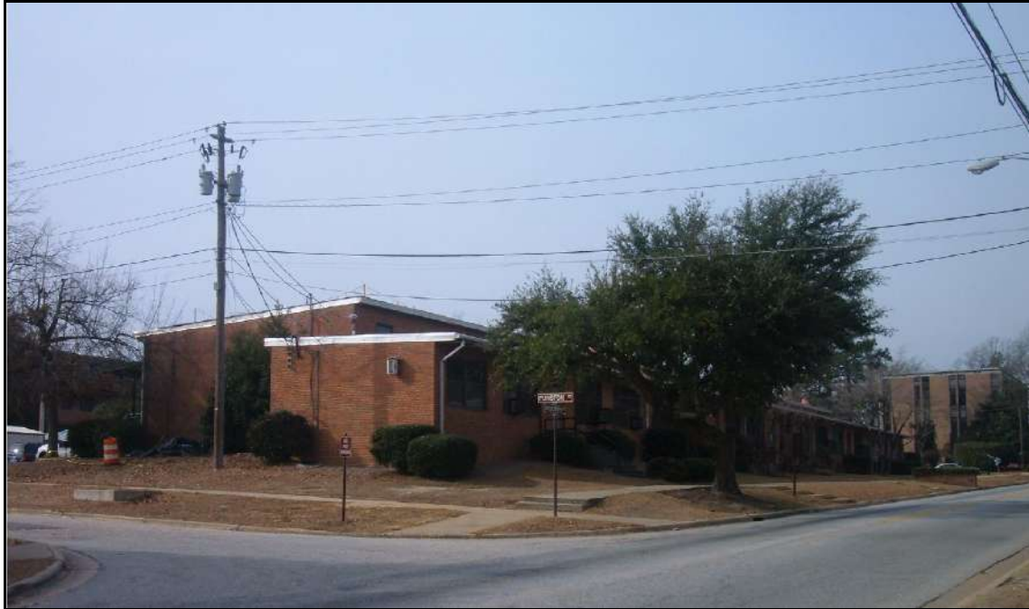
Building D-2815, north and east elevations.
