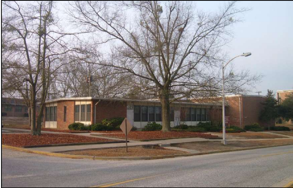
Building D-2507, north and east façades.
