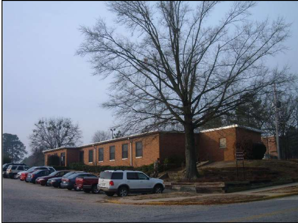
Building D-2612, north and east elevations.
