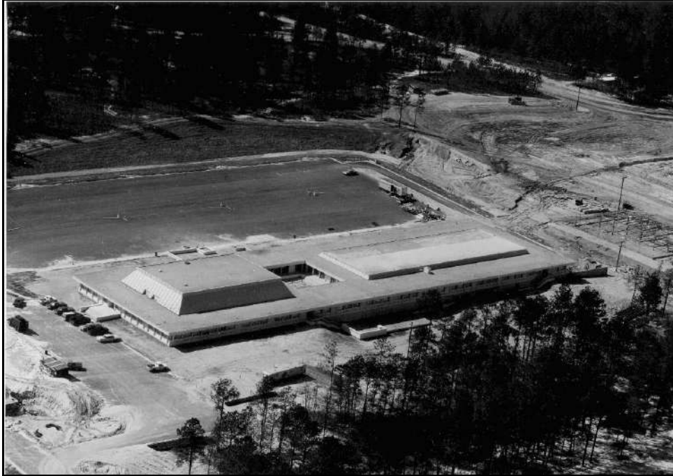
Figure 8: Kennedy Hall under construction in 1965. (Photo courtesy of the Special Operations Forces Archives)
