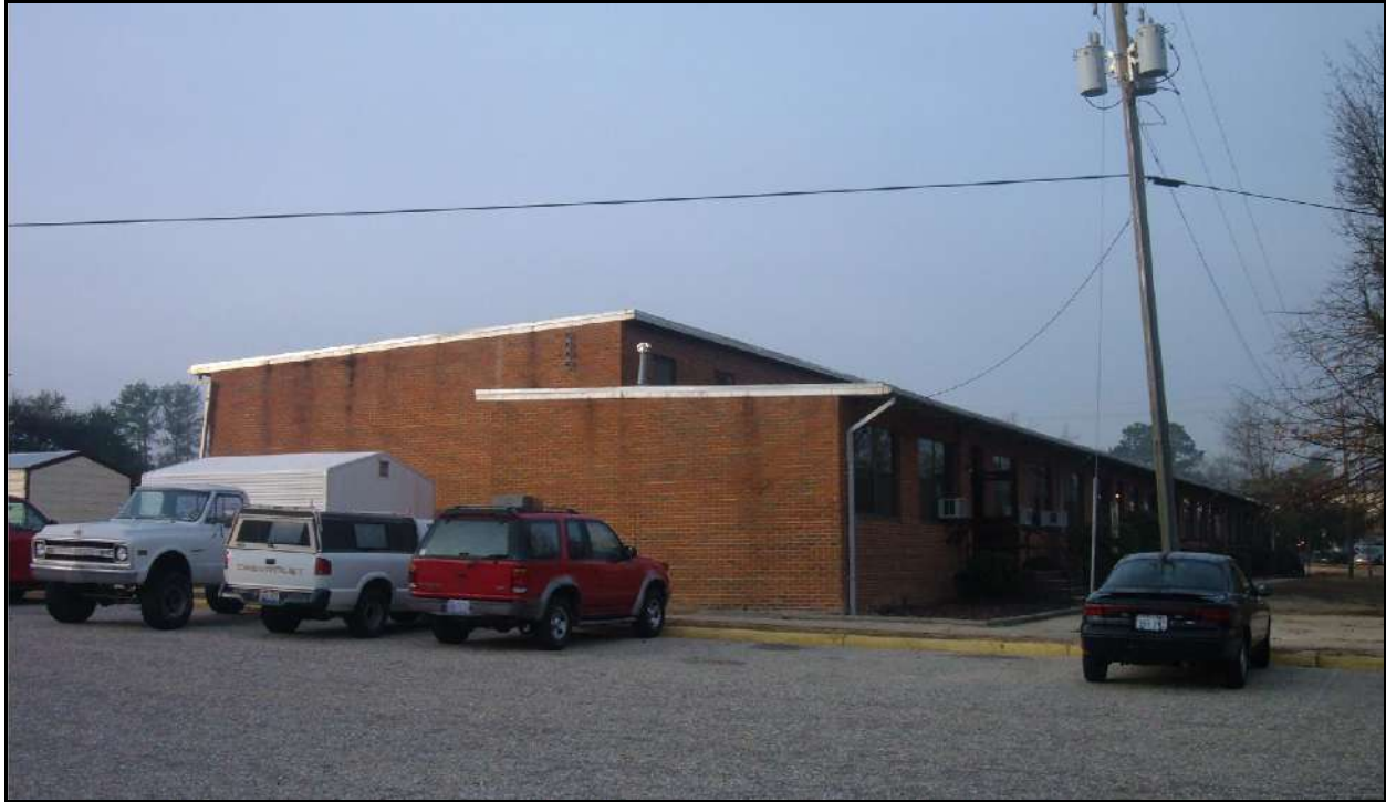
Building D-2307, north and east elevations.
