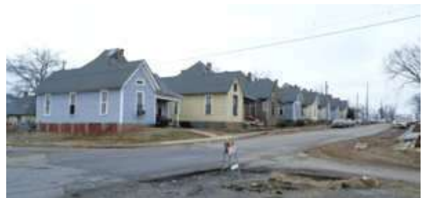
Marshall Square Historic District bounded by East 17th, South McAlmont, East 18th, and South Vance Streets 1918 solid block of vernacular rental houses Listed on 8/10/1979
