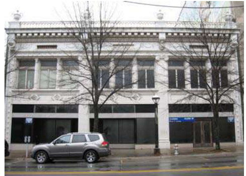
The Rose Building at 307-311 S. Main Street was an early federal tax certification project.
