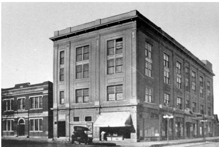
Built in 1911, the headquarters of the Mosaic Templars of America was one of the most significant buildings in Little Rock's African American community during the early-20 th century. Founded in 1883, the fraternal organization provided insurance and other services to African Americans in 26 states. (Photo is from 1924.)
