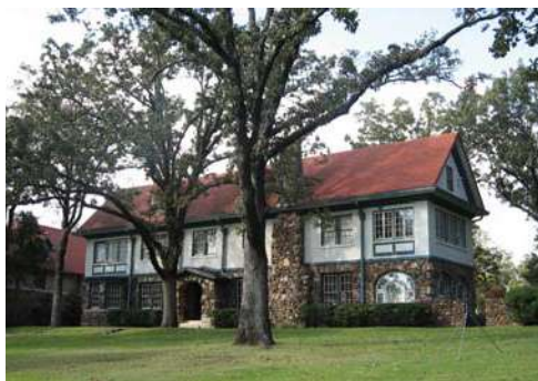
In 1992, design guidelines were prepared for the Hillcrest Neighborhood as part of revitalization efforts (3504 Hill Road).
