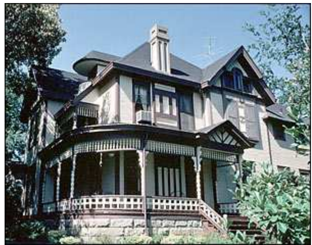
Albert Retan House 506 North Elm Street 1893 Queen Anne/Colonial Revival mix Listed on 12/3/1980
