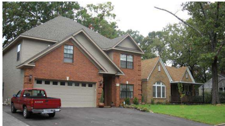
This new construction in the 1400 block of Taylor Street is out of scale and design with the adjacent dwellings in the proposed Fair Park Historic District.
