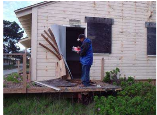
Strong enforcement measures help prevent demolition by neglect and ensuring that rehabilitation is completed in accordance with a COA.
