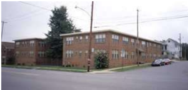
Luxor Apartments 1923 South Main Street 1924 Craftsman building Listed on 4/7/1995
