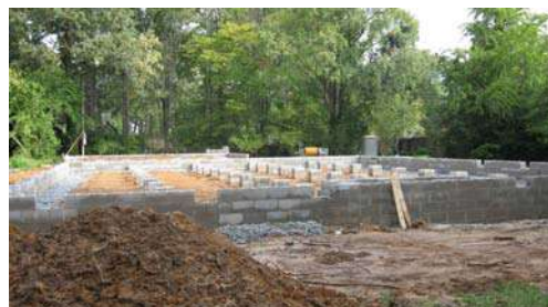
Design Overlay Districts could regulate size and scale of buildings, but not overall design (5500 block of N. Country Club Road).
