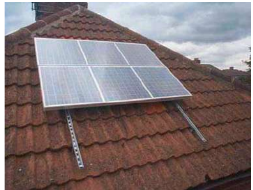
Historic dwellings can be adapted to take advantage of modern energy technology such as solar panels on rear roof lines.
