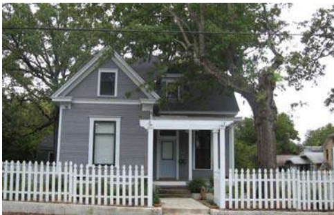
The Central High School Neighborhood is one area that has experienced significant rehabilitation efforts in recent years (1725 Park Street).
