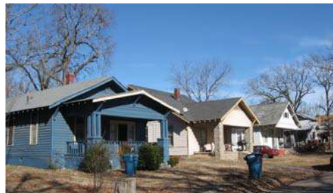
Surveys should first focus on blocks in neighborhoods developed before 1945. These have significant resources and many blocks are losing homes to abandonment and demolition (4100 block of W. 13 th Street).
