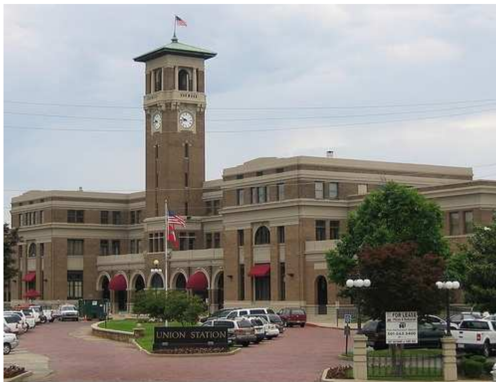
Built in 1921 at the corner of Markham and Victory Streets, Union Station provided the city with an outstanding example of Prairie architecture. It is listed on the National Register of Historic Places as Mopac Station.
