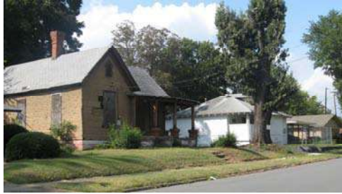
Population loss in the center-city has led to abandoned houses and deteriorated conditions on some blocks such as the 1500 block of S. Pulaski Street....
