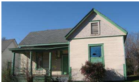
This vacant house at 918 Allis Street was built ca. 1900 and is one of many dwellings in the Stephens Neighborhood with the potential for rehabilitation.
