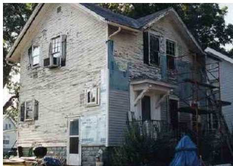
The addition of synthetic sidings such as vinyl detracts from a house's historic appearance.
