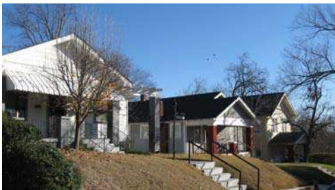
The 2900 block of S. Izard Street contains a row of frame and brick Craftsman dwellings.
