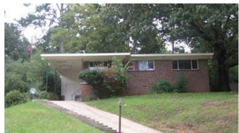
One of 18 standardized designs, this dwelling at 18 Broadmoor Drive has an attached open carport and broad hipped roof.
