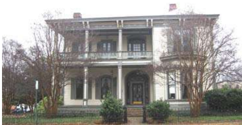
The Italianate style White-Baucom House at 201 S. Izard which was listed on the National Register in 1980.
