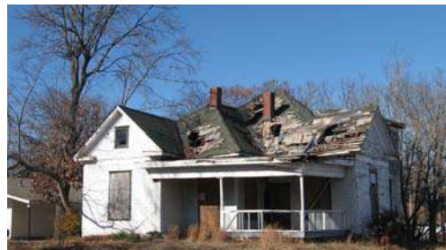
No overlay, no protection, no future. Without local ordinance districts or demolition-by-neglect provisions, this can be the result (4200 W. 16 th Street).
