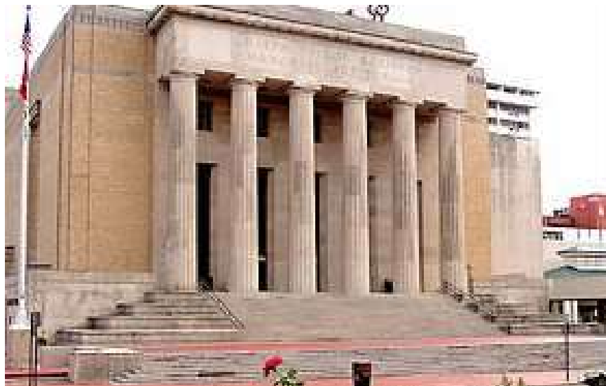
The James Taylor Robinson Municipal Auditorium, known today as Robinson Center, has been a center for Little Rock arts and culture since it was built with federal dollars as part of the New Deal of the 1930s. Its Greek Revival columns echo those found on the Old State House.
