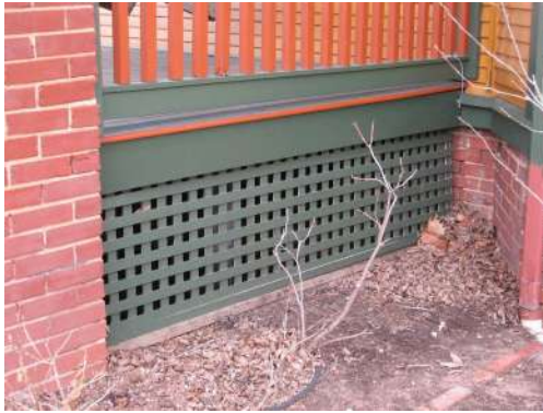
Lattice is an appropriate addition between foundation piers (left: 610 NW 17th Street, right: 2612 N. Robinson Avenue).
