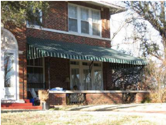
The use of canvas canopies is appropriate to provide shade for porches as at 837 NW 17th Street (left). Metal awnings such as at 301 NW 42nd Street (right) are more appropriate for rear elevations.
