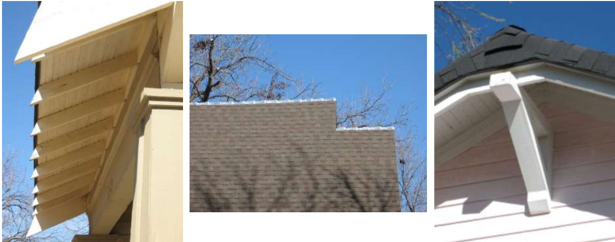
Preserve original related roof features such as rafter tails (left: 2612 N. Hudson), roof ridge tiles (center: 905 NW 38th Street), and brackets, also called knee braces (right: 1442 NW 37th Street).
