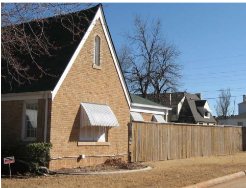
Side yard fences should have appropriate setback from the street, as at 2140 NW 26th Street.
