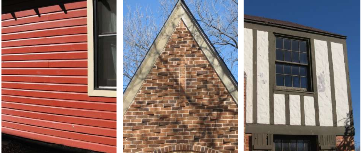
Oklahoma City's historic districts display a wide variety of original materials such as wood siding (left, 618 NW 26th Street); textured brick (center, 217 NW 31st Street); stucco and half-timbering (right, 904 NW 37th Street).
