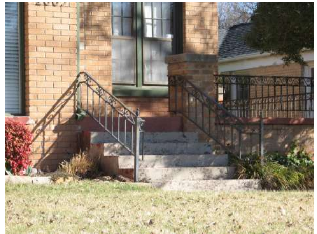
Many porch railings used for Oklahoma City's Tudor Revival style houses were built of wrought iron and these materials should be preserved and maintained. If replacement is necessary, new railings should match the original design (2133 NW 28th Street, left, and 1005 NW 38th Street, right).
