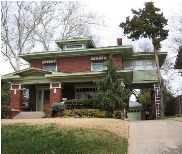
The porte-cochere at the end of the driveway at 315 NW 17th Street is an important character defining feature of the building.
