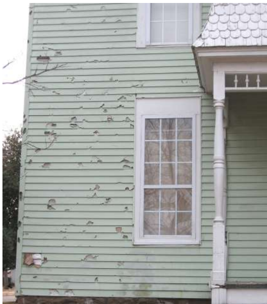
Vinyl siding is easily damaged and cannot be recycled. At left - damage caused by a hail storm.
