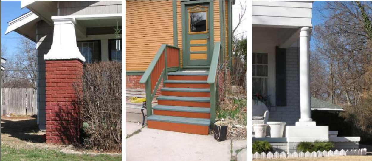
Porch components such as columns and railings are important character-defining features. These elements may be simple in design (typical in Folk Victorian dwelling), more ornate as in Queen Anne styles, or articulated as in Arts & Crafts dwellings: left, 605 NW 26th Street, the tapered wood post on a square brick pier is a typical design for a Bungalow; center, stairs at 610 NW 17th Street are of appropriate design and materials; right, 1549 NW 37th Street, Colonial Revival dwelling with Tuscan porch column.
