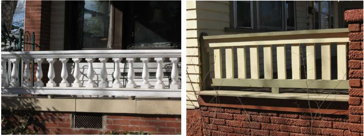
Original porch balusters (609 NW 14th Street, left, and 712 NW 24th Street, right) are character-defining and should be preserved and main-
