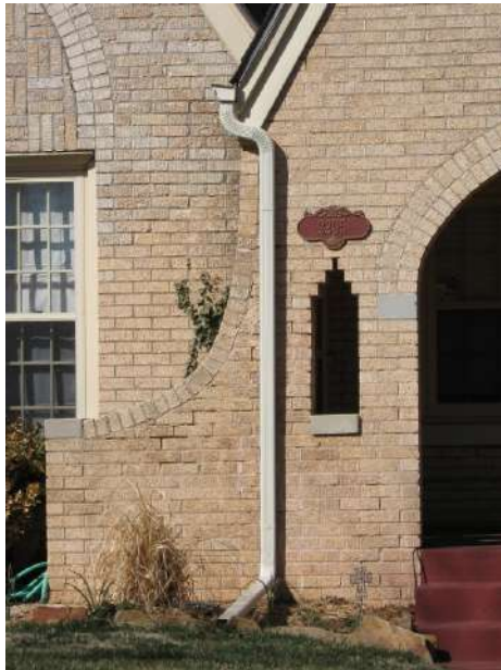
Downspouts should be located and designed to channel water away from the building (2205 NW 26th Street).
