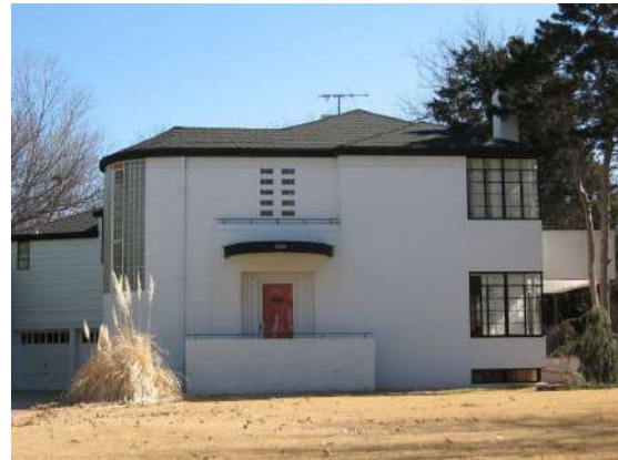
Art Moderne house at 3200 N. Harvey Parkway.
