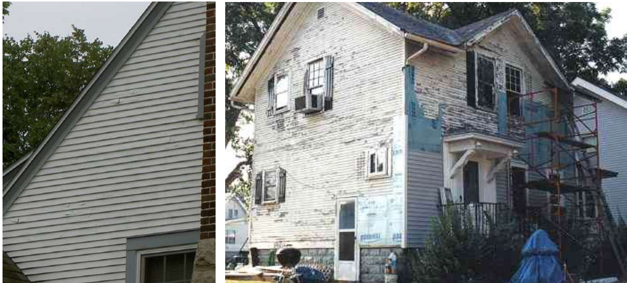
The application of vinyl siding does not allow for proper breathability of a frame dwelling and is not a sustainable material (left). After only two years, the applied polymer coating on this dwelling is already peeling (right) and the life expectancy of these materials is questionable.
