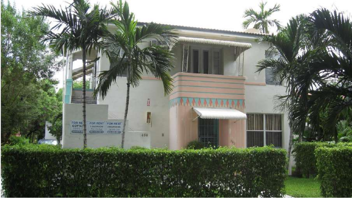
Both vertical and horizontal forms are evident on the Art Deco style dwelling at 482 59 th Street built in 1935.
