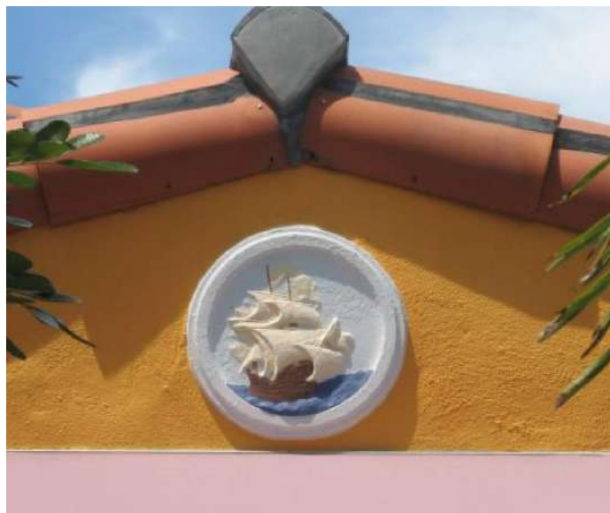
Terra cotta medallions with sea-related motifs, such as this one depicting a ship on the 1939 house at 525 72 nd Street NE, were popular ways for architects and residents to reference Palm Grove's tropical setting.
