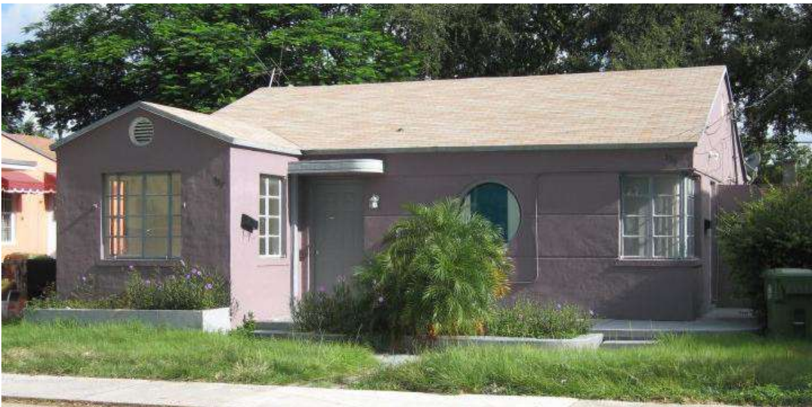
The round window, rounded-edge canopy, horizontal etched courses, and window that turns a corner all contribute to the streamlining of this 1937 duplex at 537 and 539 70 th Street NE.
