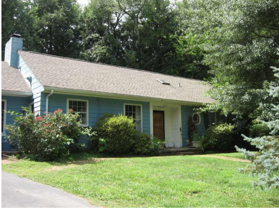
Figure 25: Fonde house with “weatherboard block” siding (KN-13343).
