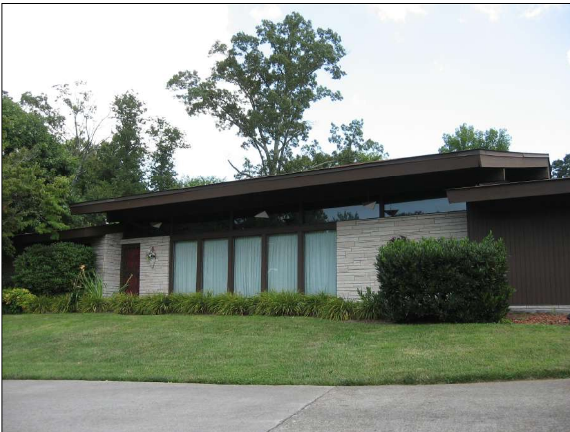
Figure 30: The dwelling at 5112 Yosemite Trail (KN-13349) features a wall of vertical fixed windows below a clerestory row of lights, accentuating the raised roofline.
