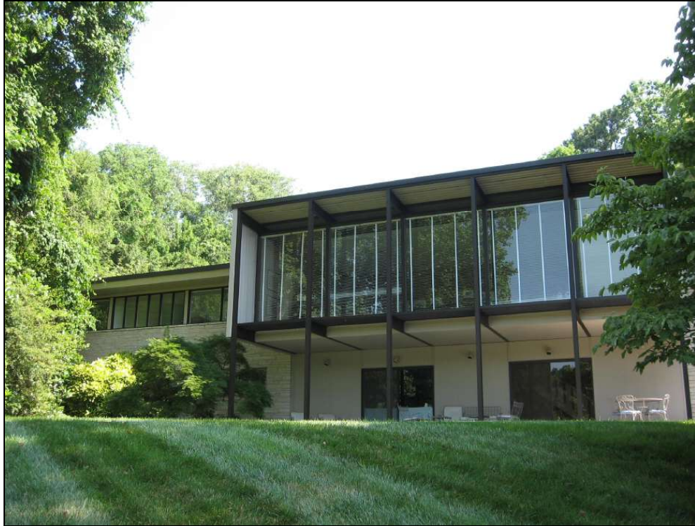
Figure 29: The cantilevered wall of glass dominates the façade of the Dr. Harry Jenkins House (KN-13329).
