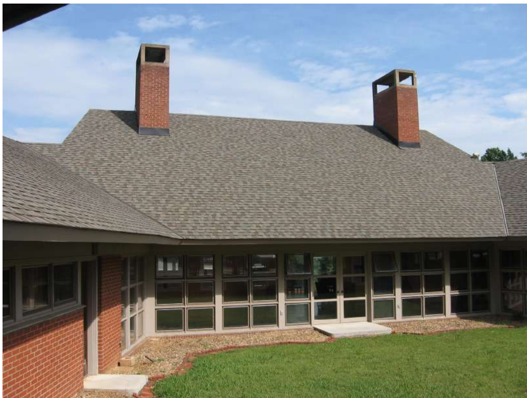
Figure 32: KN-13315 at 4703 Westover Terrace, rear elevation.
