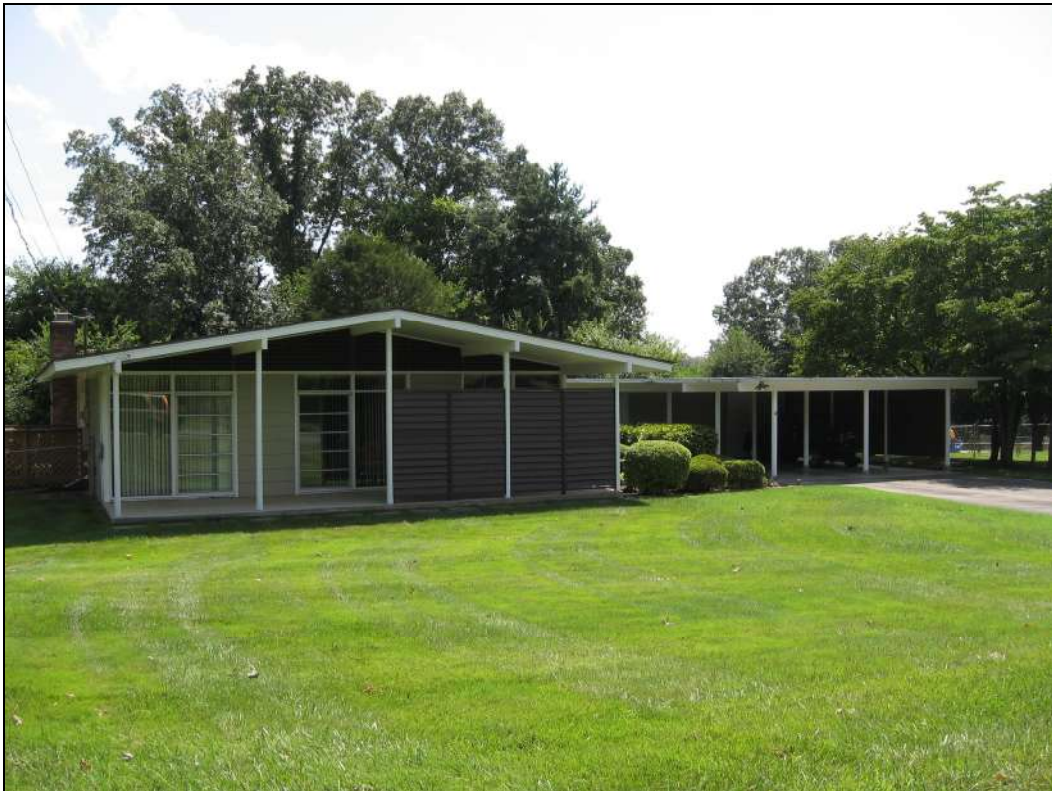
Figure 34: The dwelling at 4116 Royal View Road (KN-13350) has a side carport that leads to the main entrance.
