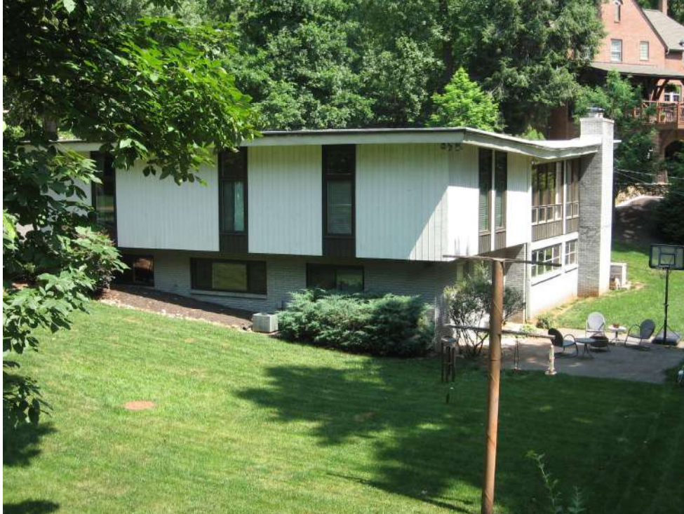
Figure 31: The dwelling at 520 Cherokee Boulevard (KN-13331) has a low-pitch butterfly roof.
