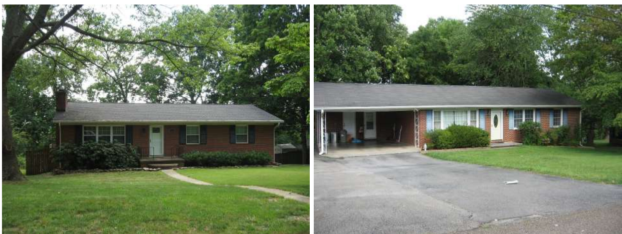
Figure 17: Examples of Inline Ranch houses at (left) 8008 West Cliff Drive and 4500 Silverhill Drive.
