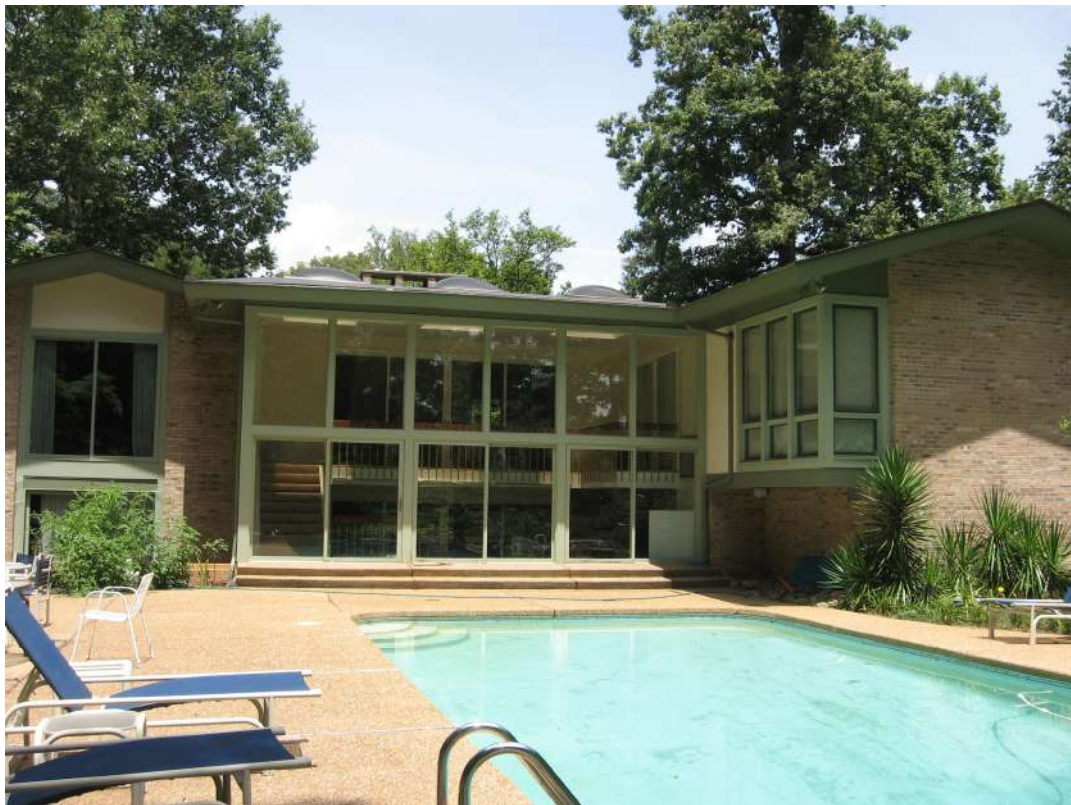
Figure 36: Rear elevation at KN-13342 at 7100 Sherwood Drive.
