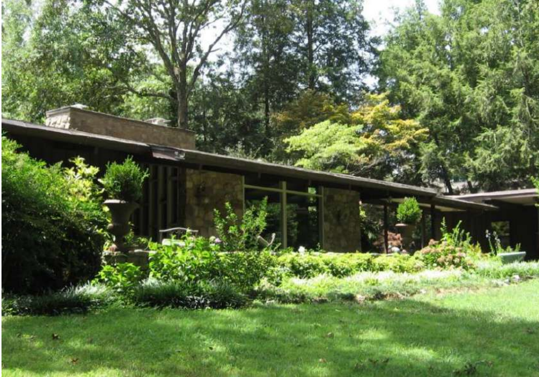
Figure 33: The dwelling at 7300 Rotherwood Drive (KN-13341).
