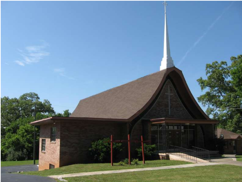
Figure 61: The Emmanuel United Presbyterian Church (KN-13321) at 3023 Selma Avenue.
