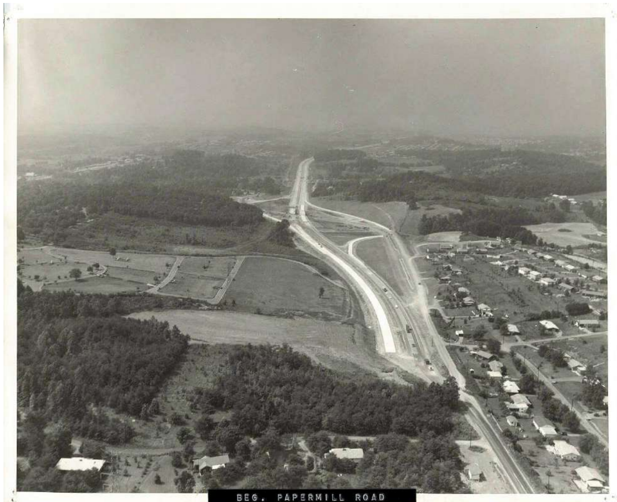
Figure 6: This view of the Papermill Road area shows the construction of Interstate 40 and new homes in the West Hills subdivision in the late 1950s (Photo courtesy McClung Library).
