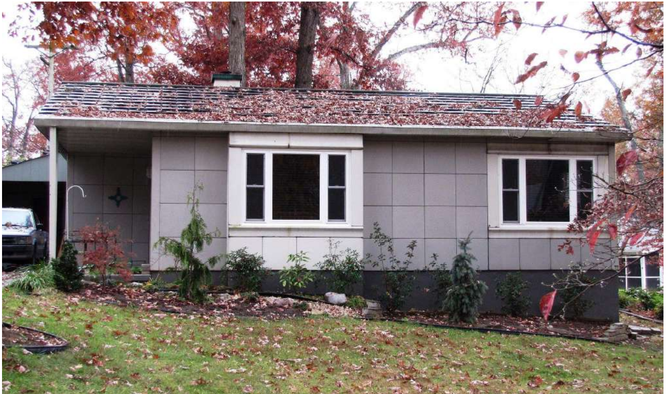
Figure 27: Lustron House at 222 Chamberlain Blvd. in Lindbergh Forest subdivision.
