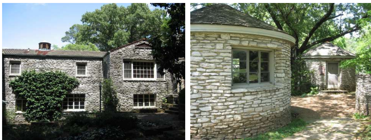
Figure 52: Howell Nursery (KN-13319) original main house and outbuildings at 2743 Wimpole Avenue.
