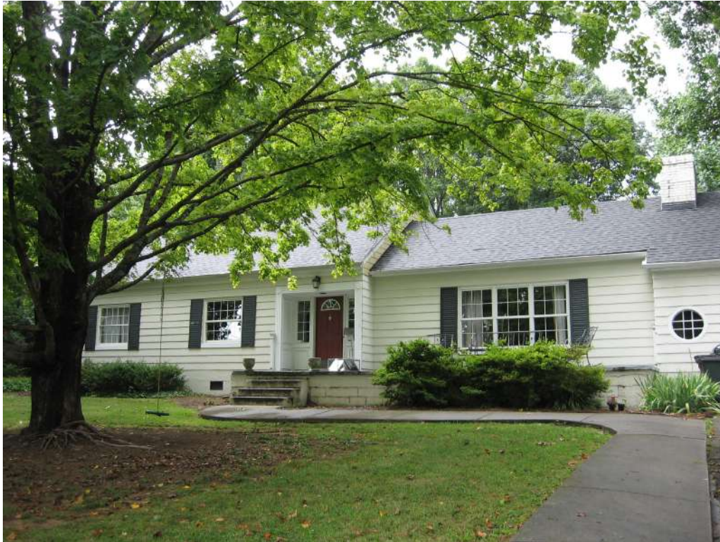
Figure 20: The house at 5901 Toole Drive is an example of Neocolonial Ranch with a recessed entrance with sidelights.
