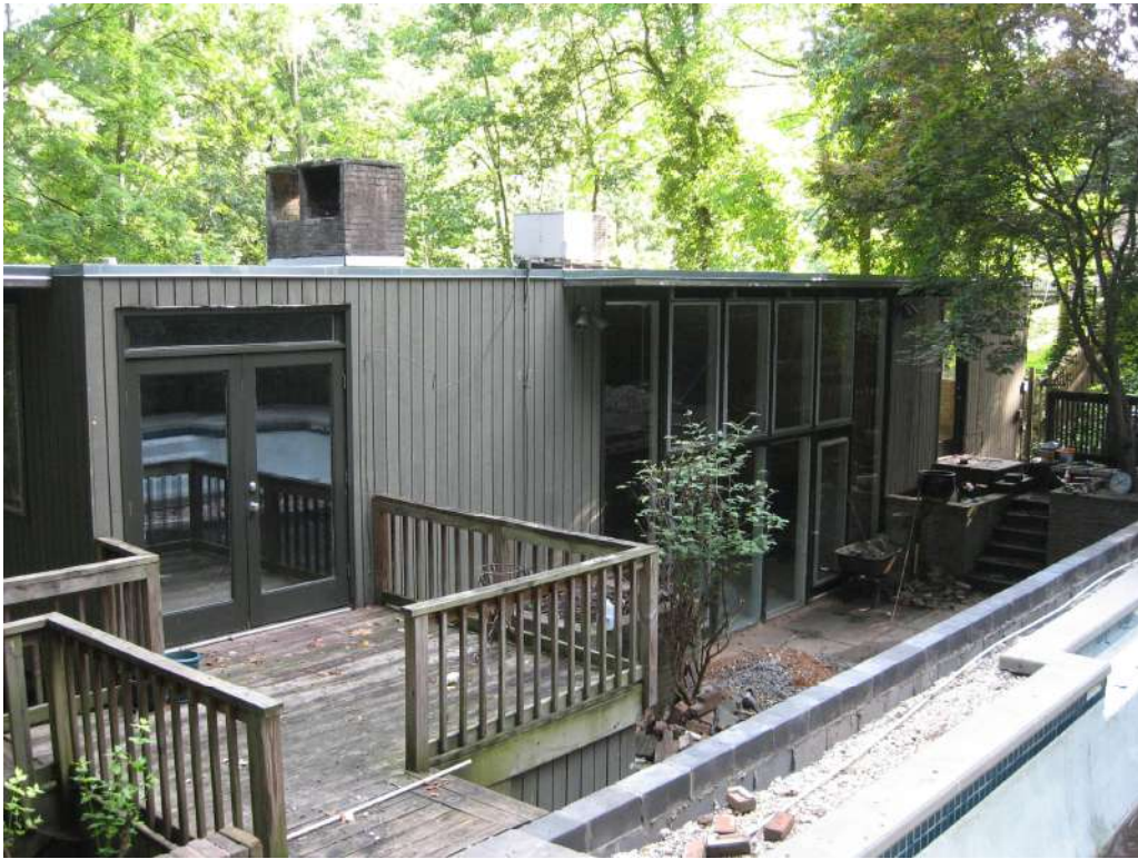
Figure 35: Rear entrances of KN-13347 at 4274 Valencia Road
