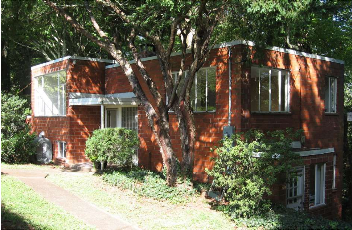
Figure 47: The Seymour House in 2016, (KN-13363).
